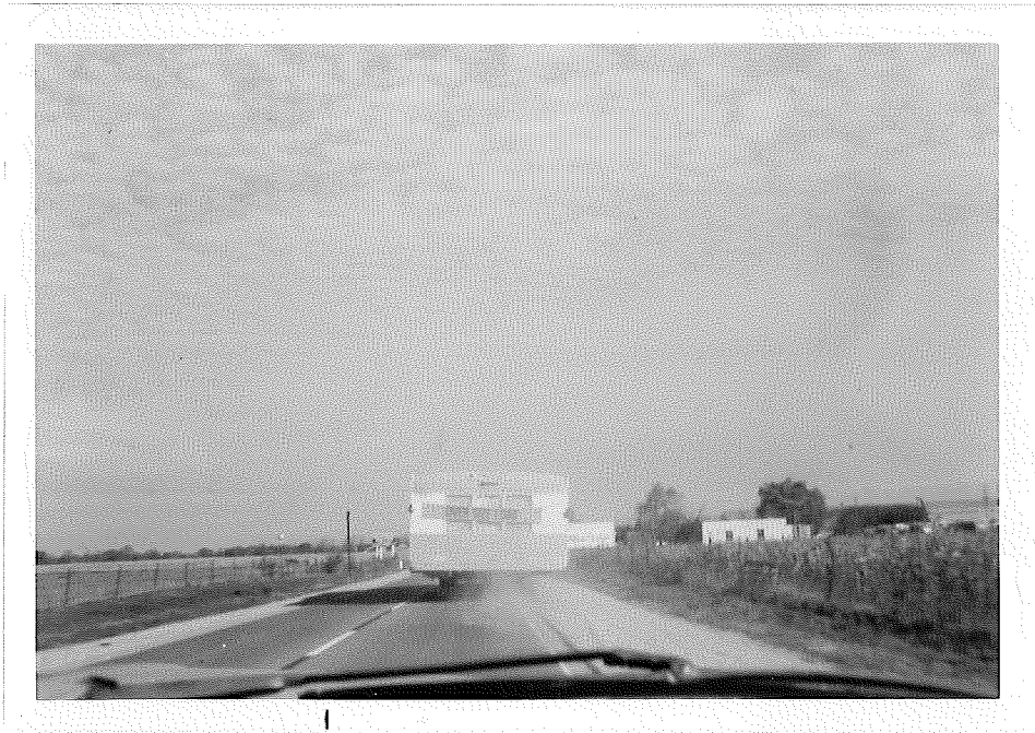
14-ft wide unit being hauled on the shoulder area blowing the clay particles from the shoulder and denoting gravel that has been thrown onto the roadway (US-131 S. of Constantine - 20-ft roadway)
