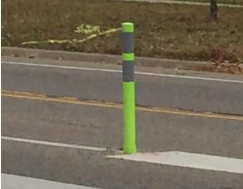
**Figure 1-4: A flexible delineator attached to a base cemented into the pavement**
