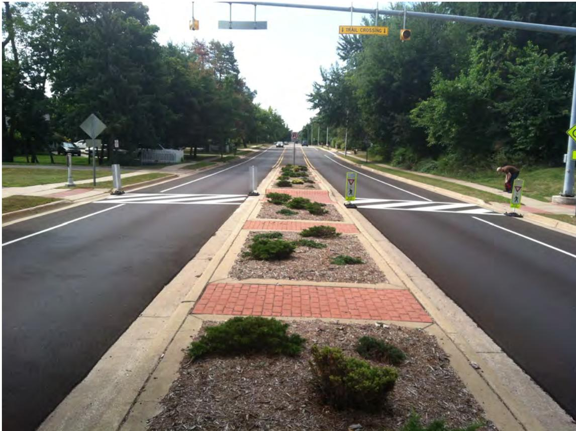
Figure 3-9. Wide gateway configuration on Oakland Street
