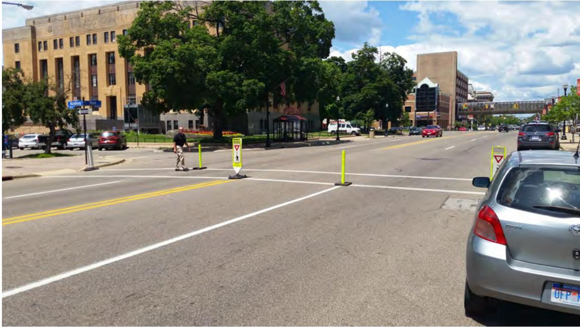
**Figure 2-6. Gateway treatment with delineators placed on white lane lines**
