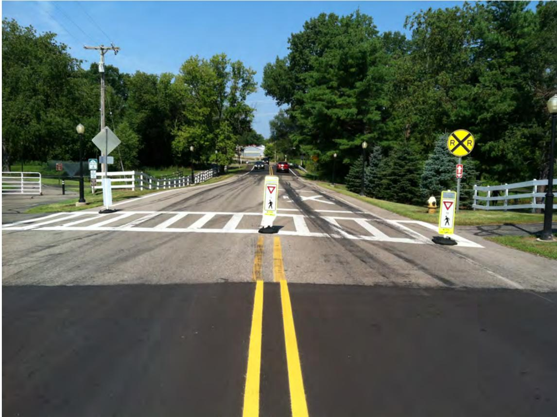
**Figure 3-10. Wide gateway configuration at the trail crossing on Garden Lane.**
