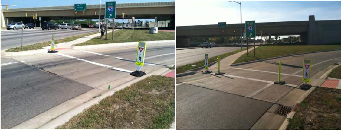
**Figure 3-7. The photo on the left shows the wide configuration of the gateway and the photo on the right shows the narrow configuration with added flexible delineator posts on the lane lines.**
