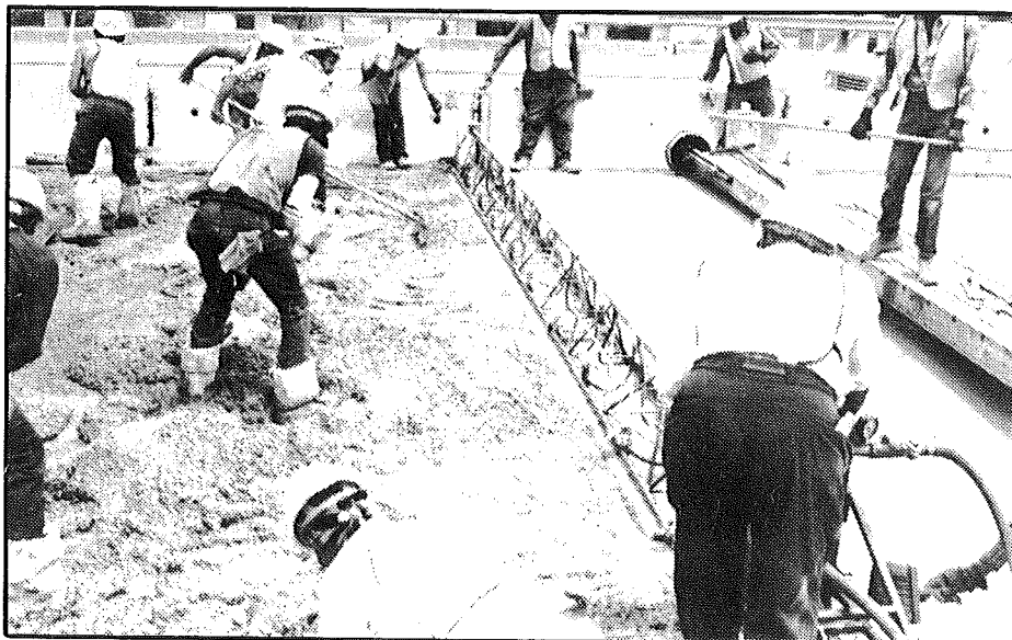
Figure 1. Placement of high density mix with superplasticizer using Allen Razorback screed on northbound I 75 (S21 of 82252).
