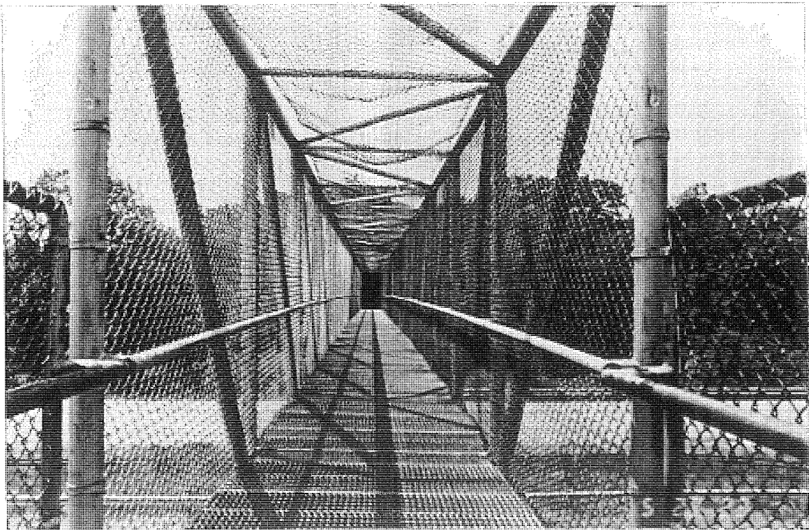
NORTH END OF DECK
