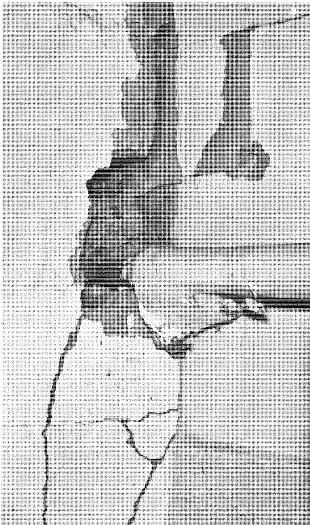
Figure 2. Condition of basement walls showing cracking at the southeast corner (upper, exterior). The center-front (left), and on the west side wall, near the southwest corner (above).
