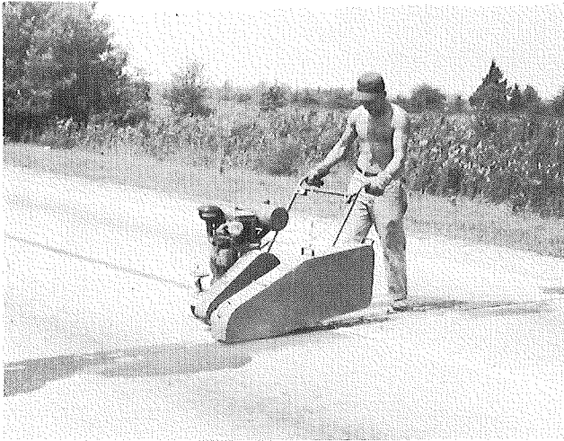
▲ FIGURE 4. HECKER JOINT CLEANING MACHINE IN OPERATION.
