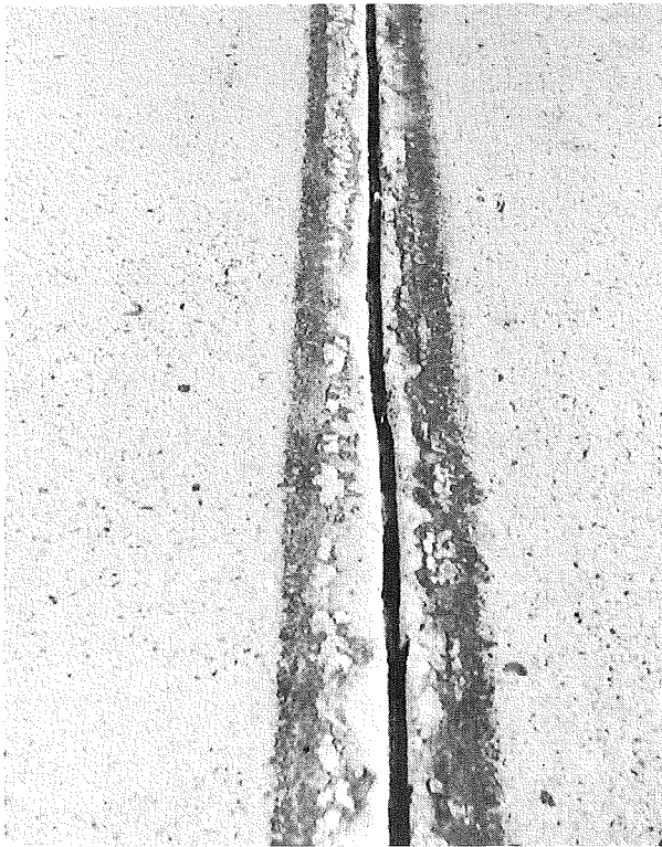
▲ FIGURE 17. CLOSEUP OF LONGITUDINAL JOINT, CLEANED AND READY FOR SEALING.
