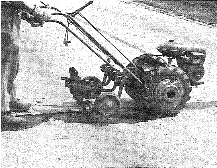
▲ FIGURE 7. GARDEN TRACTOR WITH PLOW ATTACHMENT REMOVING OLD JOINT SEALER.
