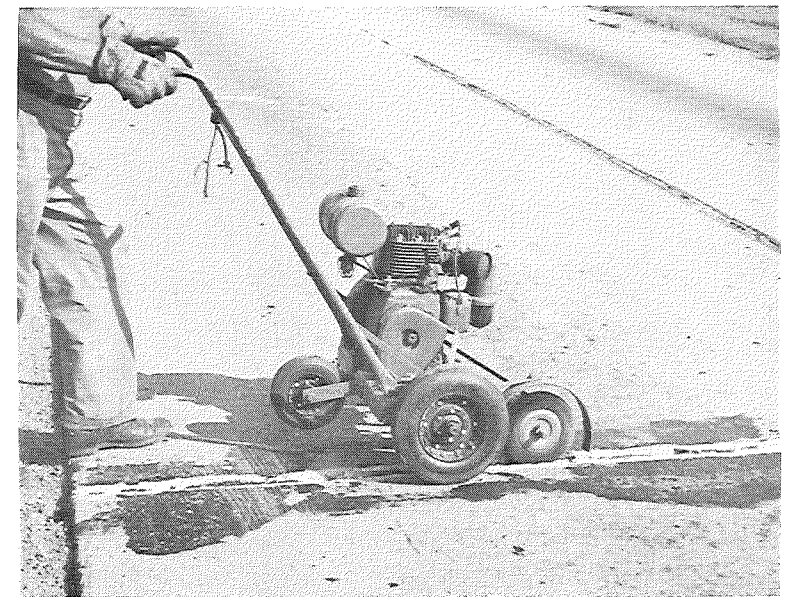
▲ FIGURE 10. MECHANICAL WIRE BRUSH USED IN EARLY JOINT CLEANING OPERATIONS.
