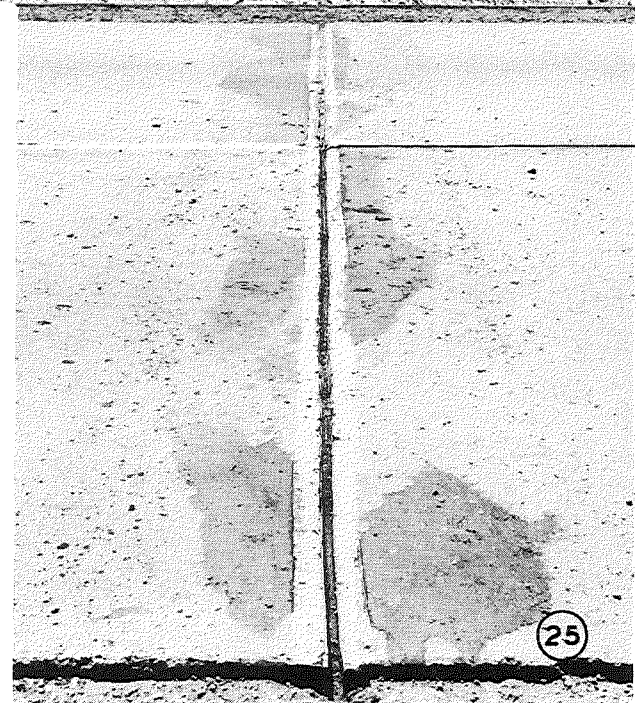
FIGURE 22. CLOSED CRACK AFTER SANDBLASTING V-SHAPE GROOVE ALONG CRACK.
