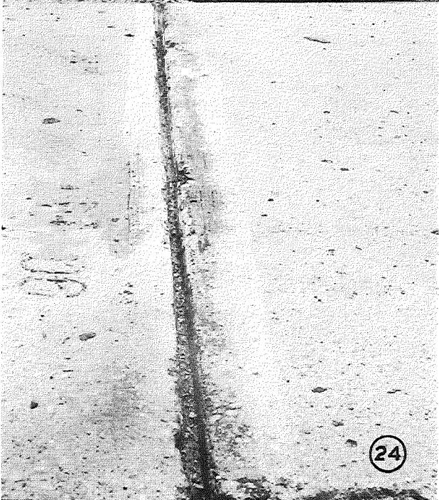
FIGURE 21. OPEN CRACK CUT OUT WITH TENNANT MACHINE, READY FOR SEALING.
