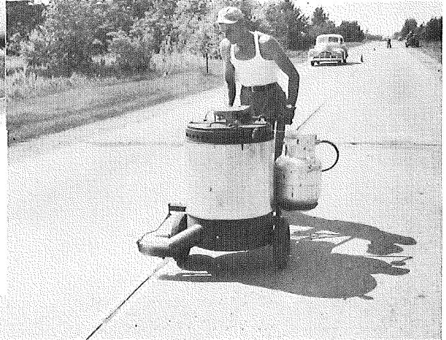
▲ FIGURE 3. USE OF MECHANICAL POUR POT IN SEALING LONGITUDINAL CENTER JOINT.
