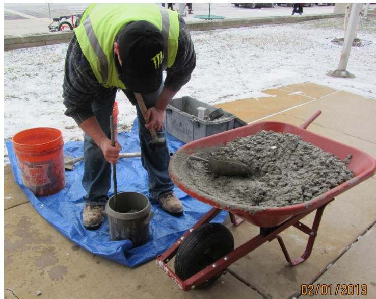
Figure 5.2.3 – Fresh concrete onsite testing
