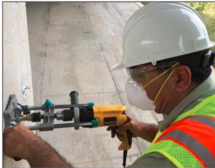
Figure 6.6 – Coring around dollies for proper adhesive bond testing
