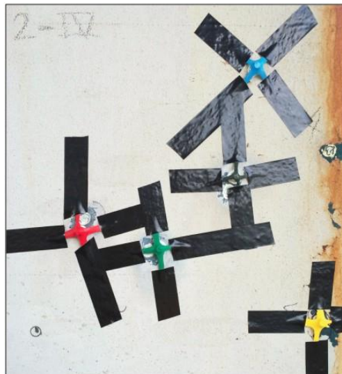
Figure 6.4 - Test dollies installed on column 2, face 4
