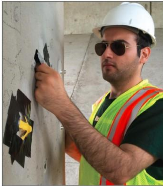
Figure 6.5 – Removal of tape and elastic membrane to expose dollies for testing
