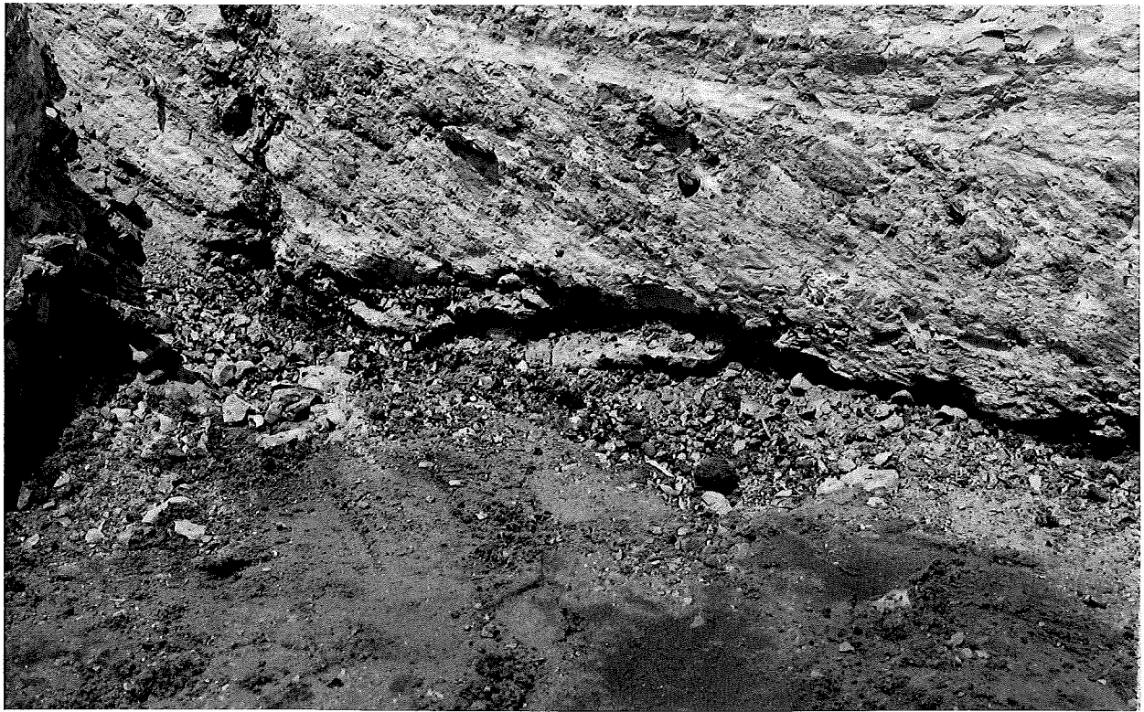
Figure 4. Ledges or "stepping" in vertical edge near centerline of the pavement.
