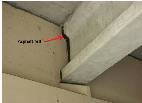
Figure 6-3. Pier-diaphragm-beam end connection details
