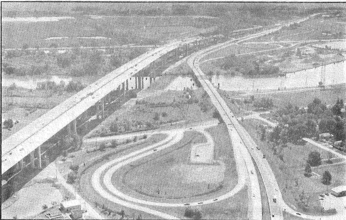
Figure 1. The nearly completed Zilwaukee Bridge and the existing bascule bridge it will replace.
