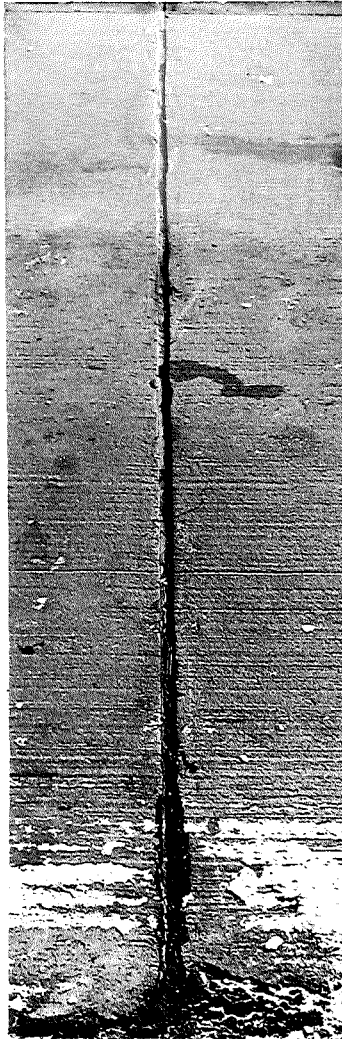
Figure 2. Polysulfide two-component sealer (Presstite) gave satisfactory performance after three month's service; Sta 670+95 (SB).
