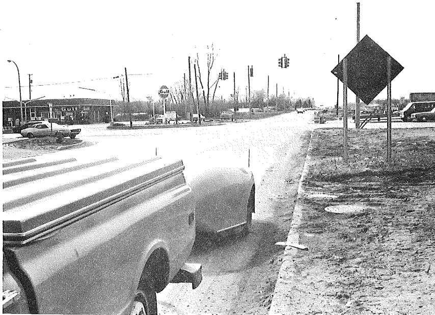
Schoolcraft Road - Soil from construction operation on pavement.
