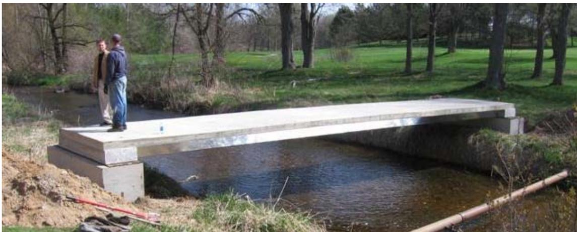
**Figure 11. Pedestrian Bridge over Tyler Creek (MI) with Cons-Struct System (Nelson, 2006)**
