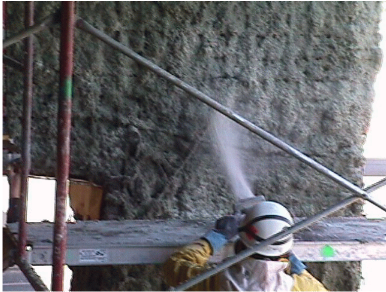
Figure 3 Application of Cellulose Fiber Mix.
