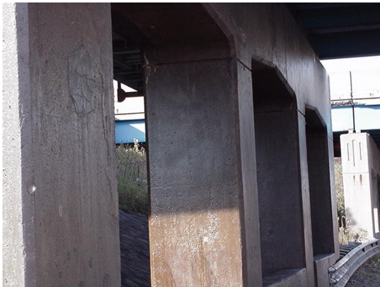
Figure 10 ECE Treated Pier with penetrating sealants applied.
