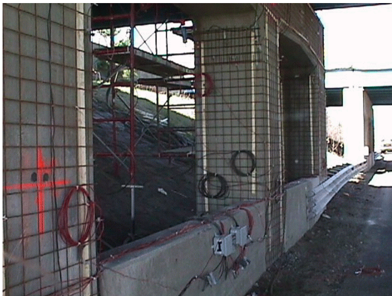
Figure 2 Installation of the Anode Mesh
