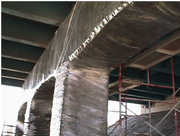
Figure 4 Plastic Wrap to keep cellulose fibers moist.
