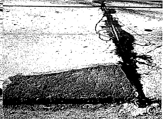
▲ STATION 463 +63. A SINGLE CORNER BREAK REPAIR.
