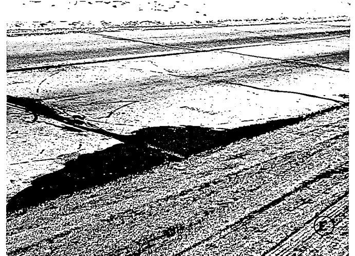
GENERAL VIEW OF REPAIR SHOWN IN D. ▶
