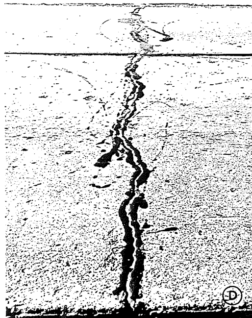
◀ STATION 454 +61. SEALED WITH BRAND E. PERFECT SEAL HAS BEEN MAINTAINED.
