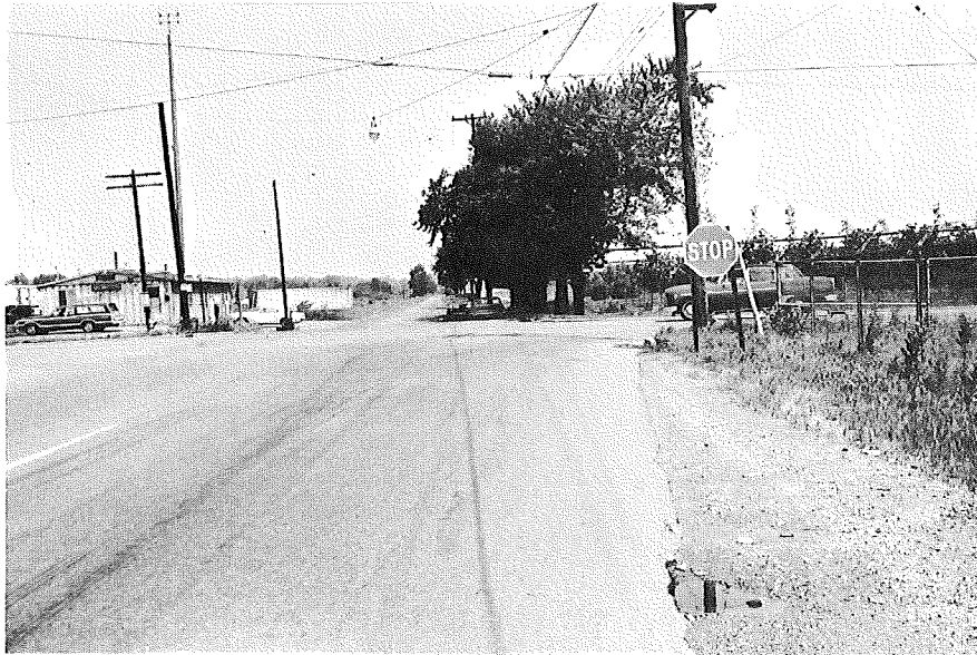
NORTHBOUND PITCHER ROAD
