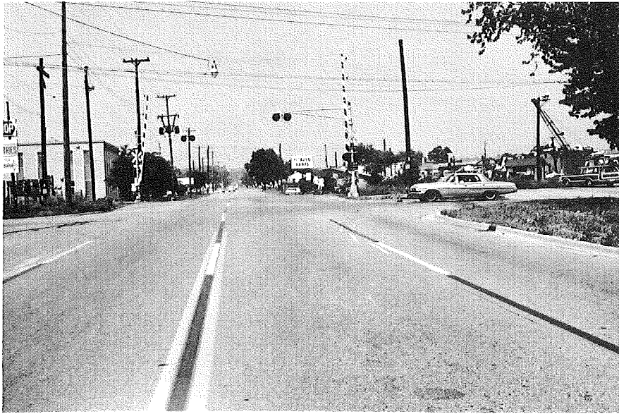
WESTBOUND MOSEL AVENUE
