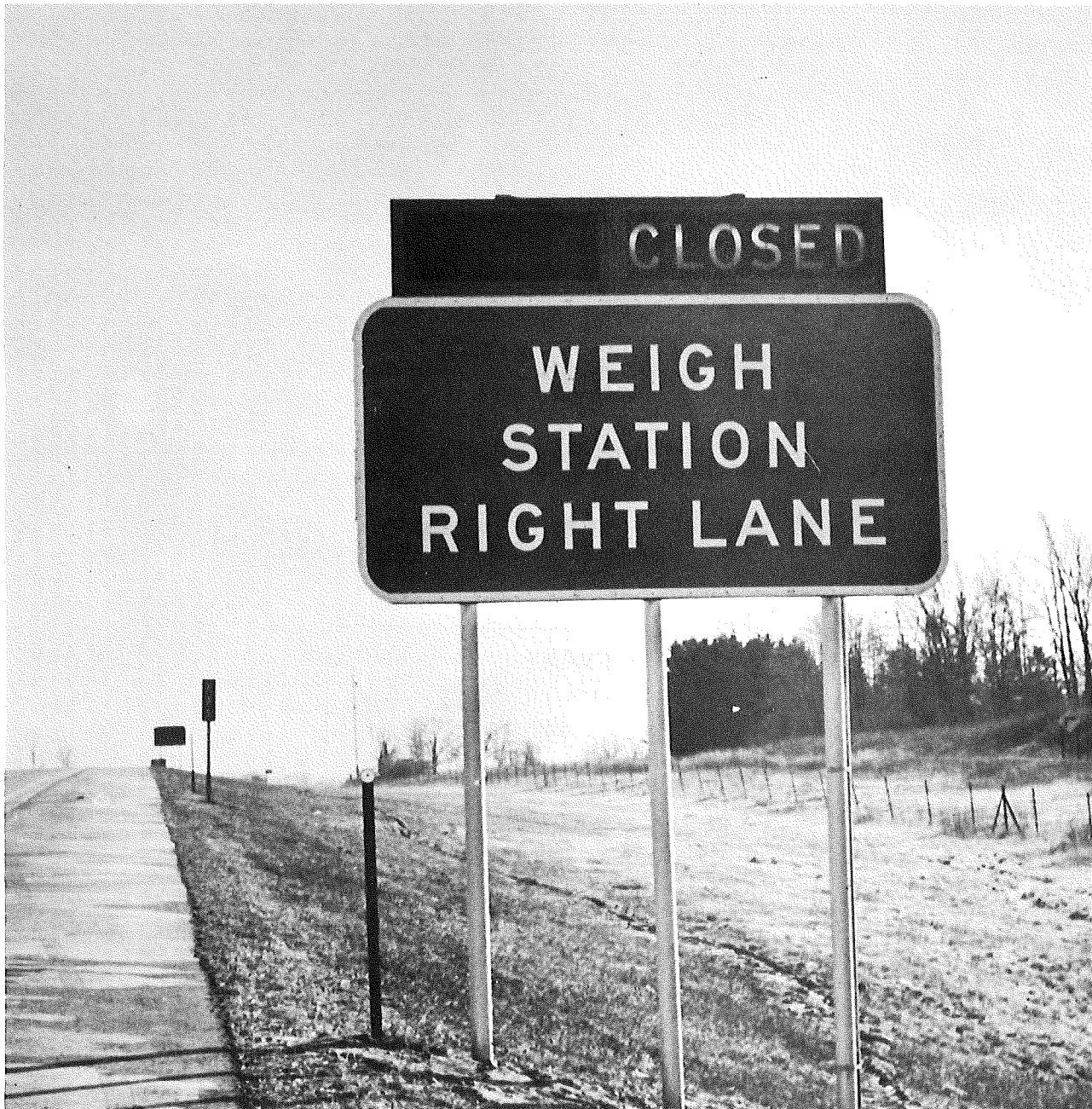
PHOTOGRAPH #4 - FLUORESCENT TYPE SIGN TO AASHO REQUIREMENTS AS USED IN FIELD STUDY
