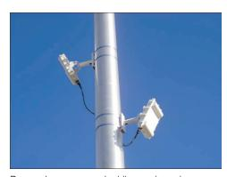
Researchers proposed adding nonintrusive MVDS sensors (shown here on roadside poles) to MDOT's traffic monitoring network to improve coverage while reducing installation and maintenance costs.
