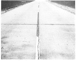
Broom finish, cutback asphalt curing Section 2B, Sta. 620+00
