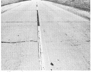
Natural cement without grinding aid Section 6A, Sta. 584+80
