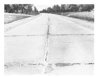
Broom finish, wet straw curing Section 1B, Sta. 377+10
