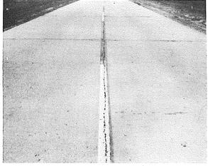
Broom finish, wet earth curing Section 1B-1, Sta. 625+00
