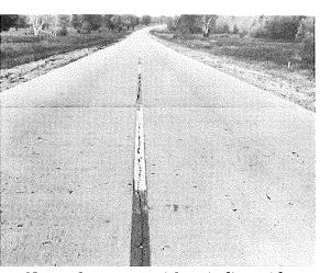
Natural cement with grinding aid Section 6C, Sta. 609+00
