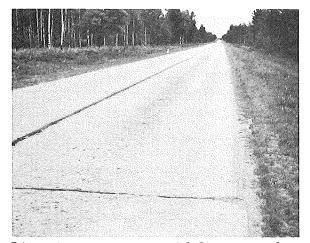
Limestone aggregate with limestone dust (May 1951) Section 8A, Sta. 753+46
