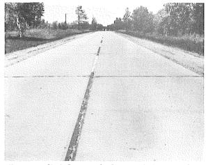
Broom finish, asphalt emulsion curing Section 2A, Sta. 384+00
