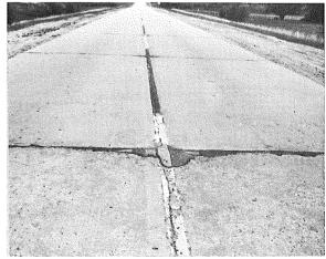
Standard construction, Cement No. 1 Construction joint in foreground Section 6B, Sta. 599+15
