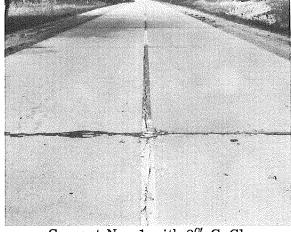
Cement No. 1 with 2% CaCl<sub>2</sub> Section 4A-1, Sta. 412+40
