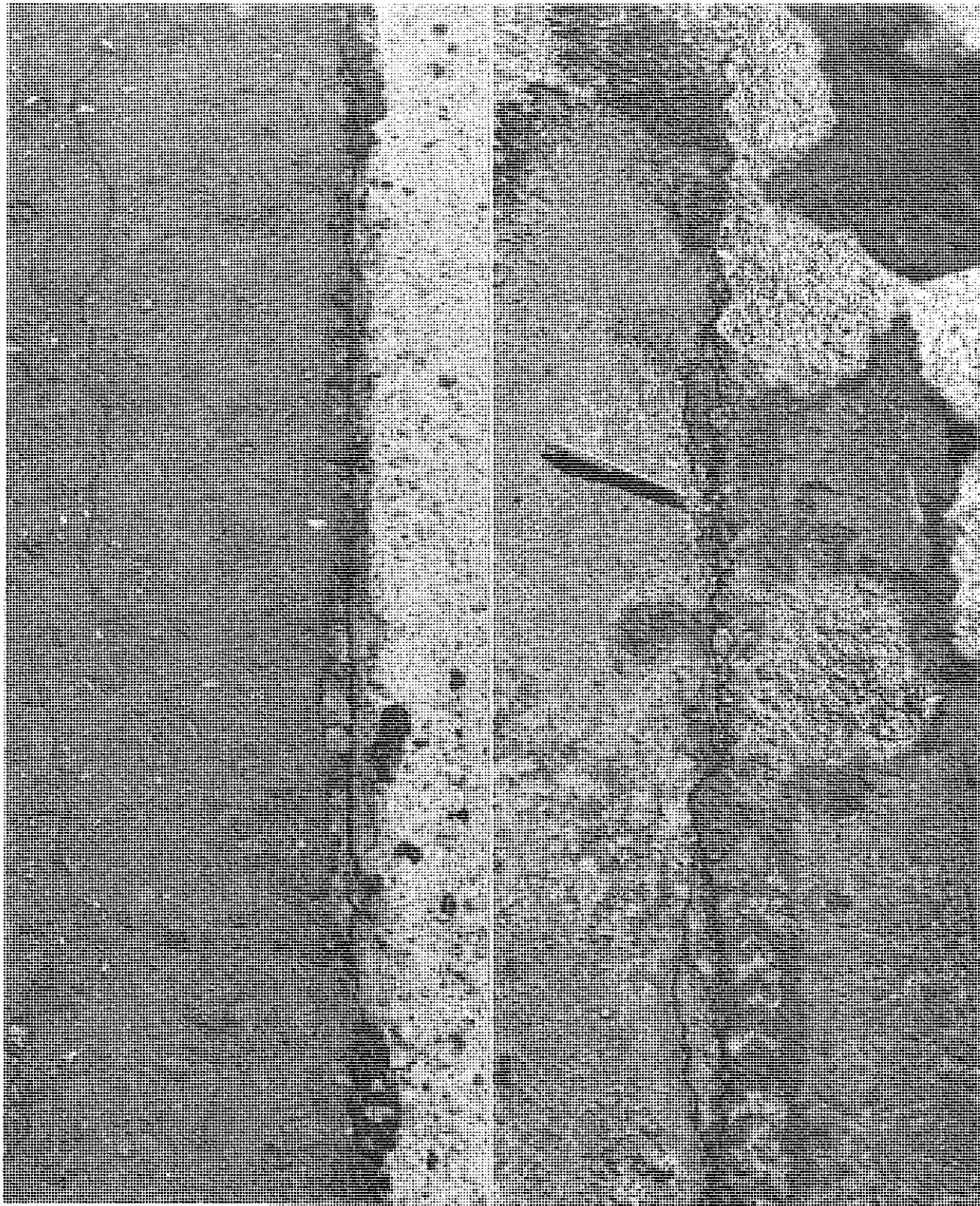
Sta. 1064+00 Project 1: EB Roadway Age: 11 months
