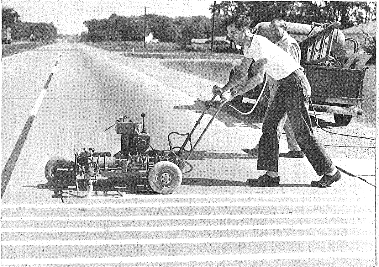
Figure 2, Paint Striping Machine in Operation
