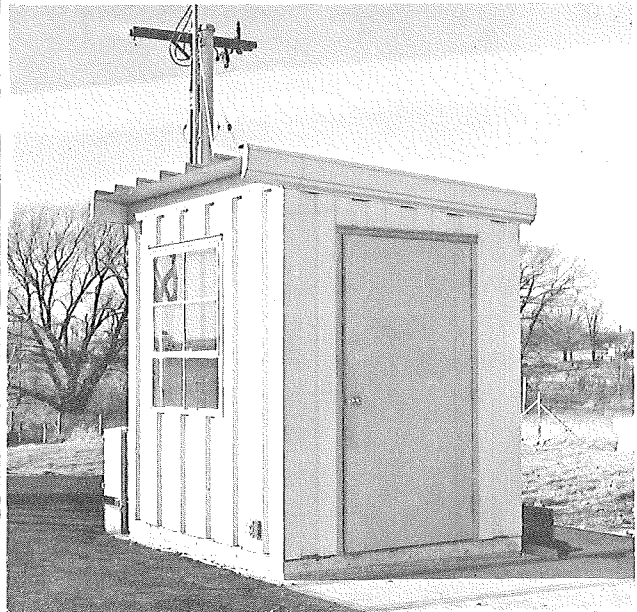
Figure 6. Shoulder enclosure serving as the junction and distribution point for all evaluation path power and signal circuits, and containing power supplies, amplifiers, and system preprocessing equipment.
