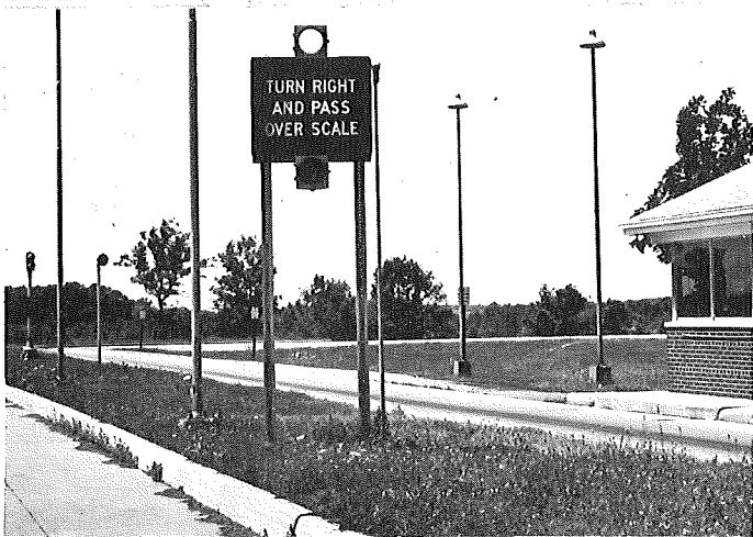
▲ Should a vehicle found to be illegal take the bypass lane in violation of the overhead sign directions it would be presented with this flashing message to take the turn-off, circle around behind the scalehouse and then enter the scalehouse lane and stop on the mechanical scale (no message is visible when the sign is not illuminated).
