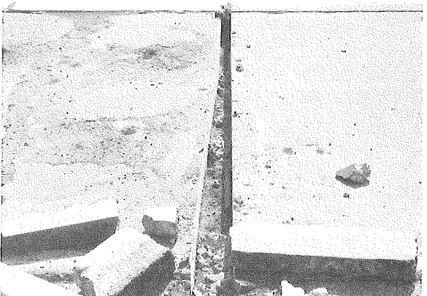
Figure 6b. The concrete between the double saw cuts has been removed to relieve compression in the slab. ▶
