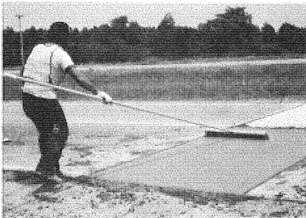
▶ Figure 24b. Prior to the concrete gaining its initial set, the groove forming strips are removed.
