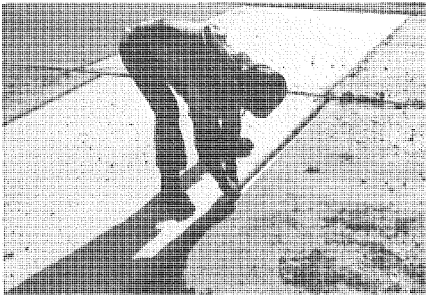
Figure 27b. A tape is installed in the bottom of contraction joint grooves to prevent the sealant from bonding to the bottom of the groove.
