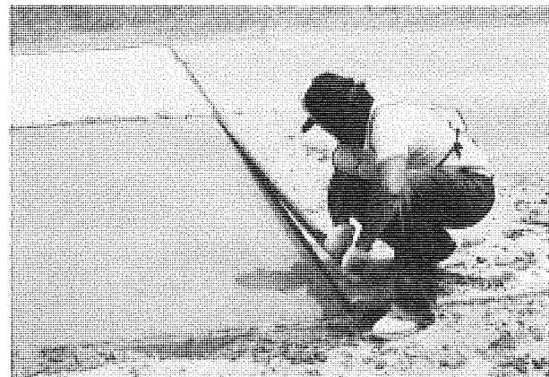
▶ Figure 24b. Prior to the concrete gaining its initial set, the groove forming strips are removed.
