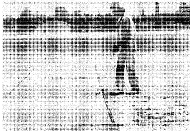
◀ Figure 23b. The surface is textured by using a coarse broom.
