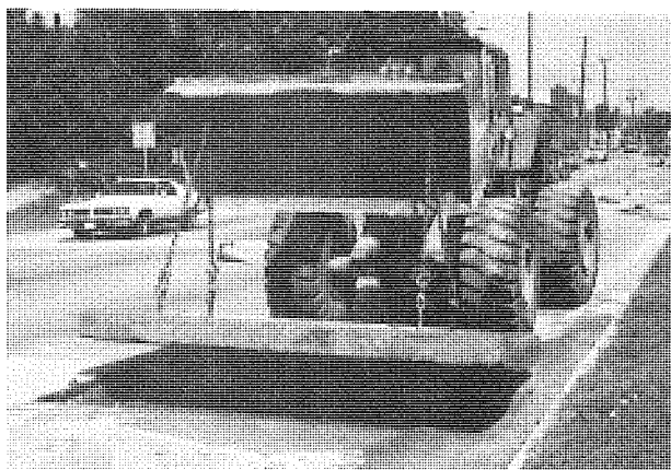
Figure 9b. The broken concrete pieces are loaded on a truck and transported to disposal site.
