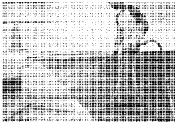
Figure 12b. Dowel holes are cleaned by using compressed air.
