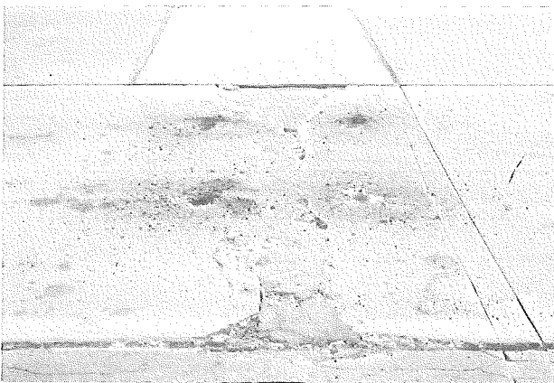
Figure 6b. The concrete between the double saw cuts has been removed to relieve compression in the slab. ▶
