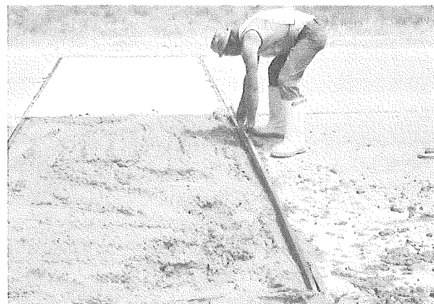
◀ Figure 17b. The replacement concrete must meet the specified slump requirement to ensure that the strength can be obtained within the specified time limit.
