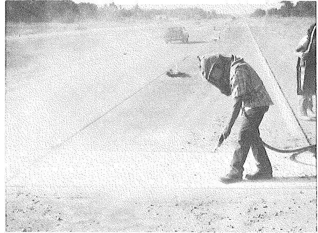
Figure 27b. A tape is installed in the bottom of contraction joint grooves to prevent the sealant from bonding to the bottom of the groove.
