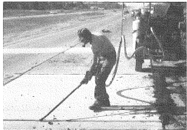
Figure 27b. A tape is installed in the bottom of contraction joint grooves to prevent the sealant from bonding to the bottom of the groove.
