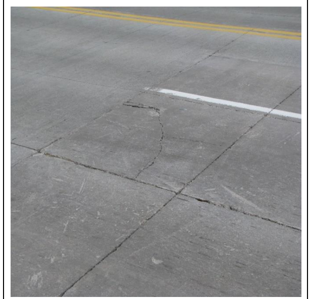
Figure 6. Distress Slabs South of Pinconning Bridge on M-13
