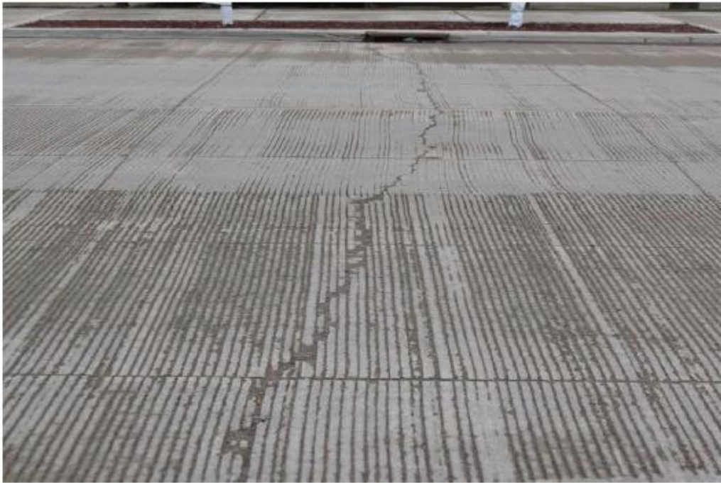
Transverse crack 90 from POE, NB-1
