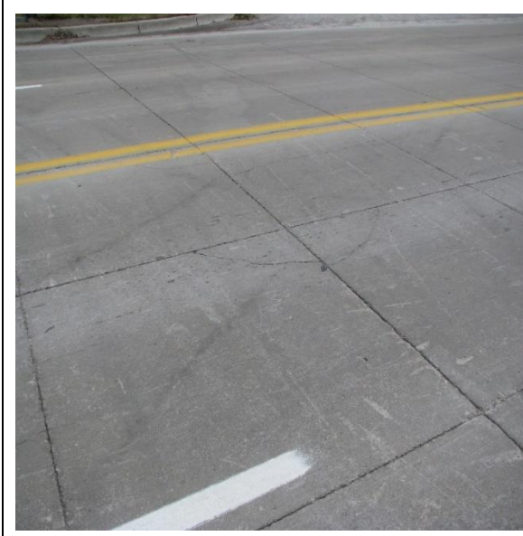
Figure 6. Distress Slabs South of Pinconning Bridge on M-13
