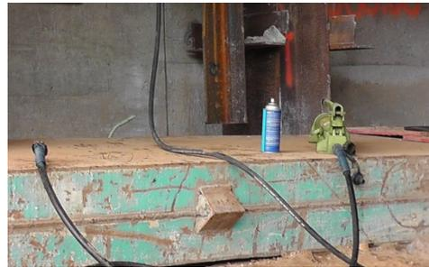
**Figure 1-6 Manual jack at fascia girder and pump**
