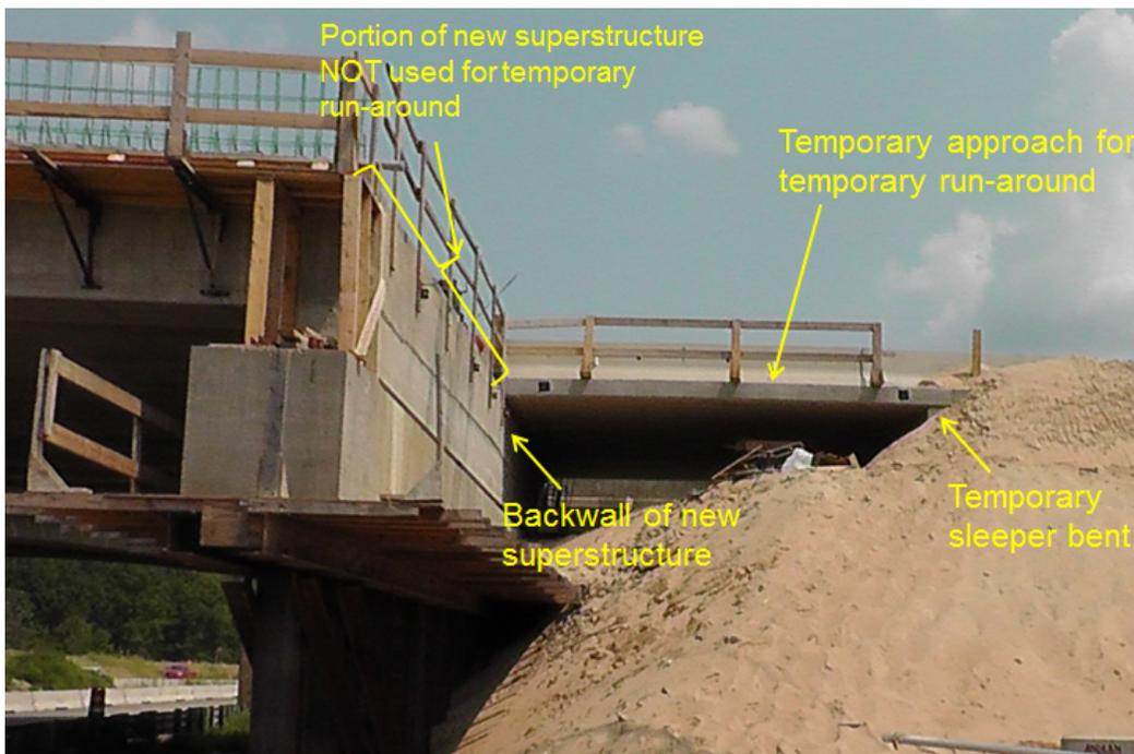
Figure 1–12 New superstructure at temporary location with temporary run-around in-place
