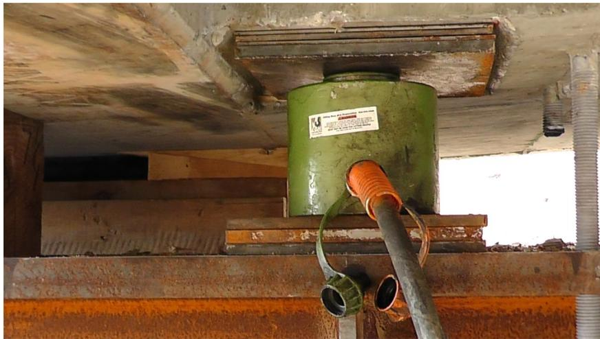
**Figure 1-4 Jack with 100 T capacity at the backwall pocket**
