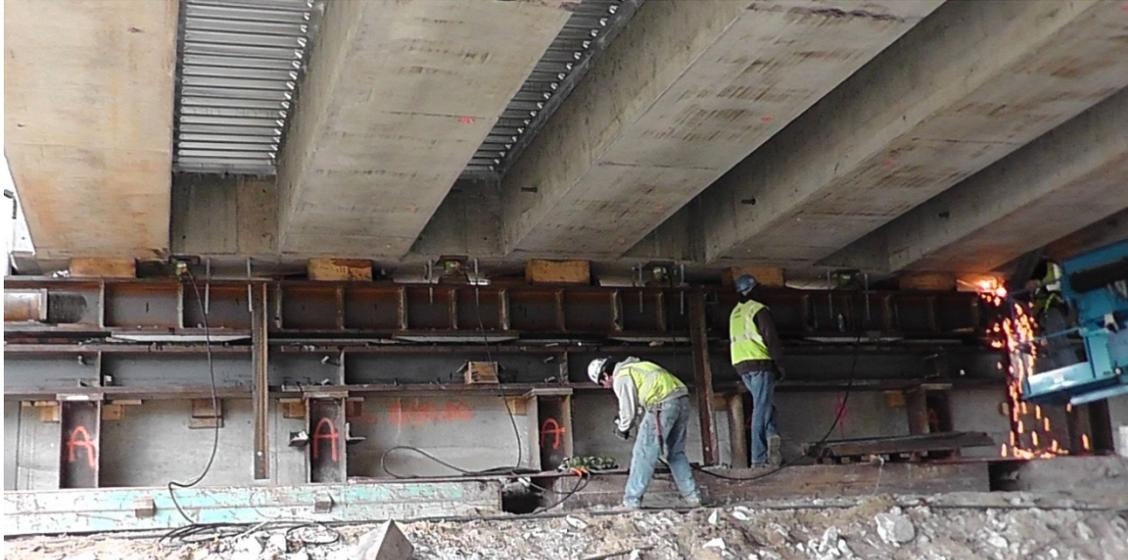
**Figure 1-3 Synchronized jacks at the backwall pockets**
