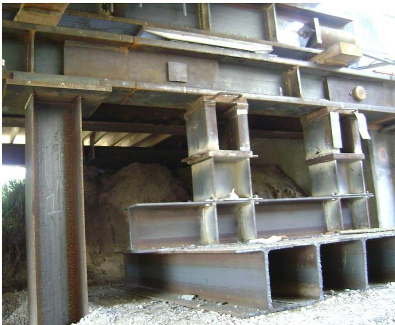
**Figure 2-4 Additional temporary supports at the transition zone for NB superstructure**
