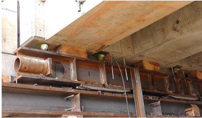
**Figure 1-5 Manual jack under the fascia girder**
