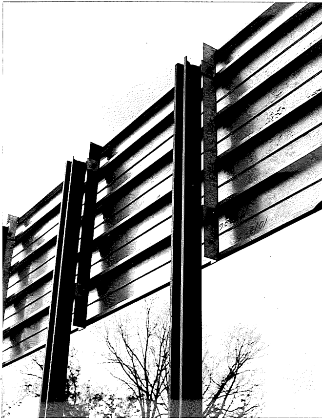
Figure 5. Three-post sign support assembly on eastbound I 96 (legend: "Detroit 39"). Steel members are in direct contact with aluminum, and corrosion has begun. Age: 3 months.
