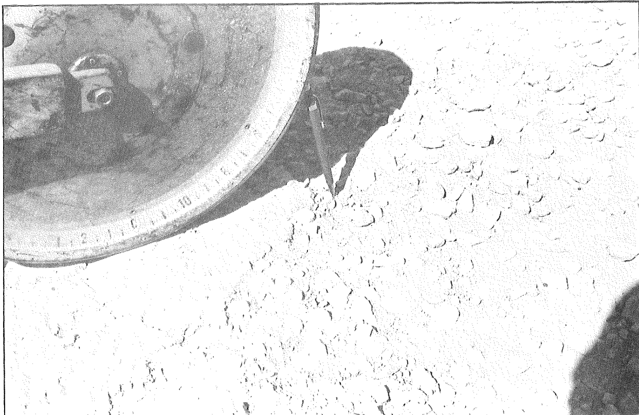
Figure 4. Loss of a thin layer of material from top surface of LFA base course is shown in the upper photo. Loss of approximately 3/4 in. of material from top surface of LFA base course is shown below.
