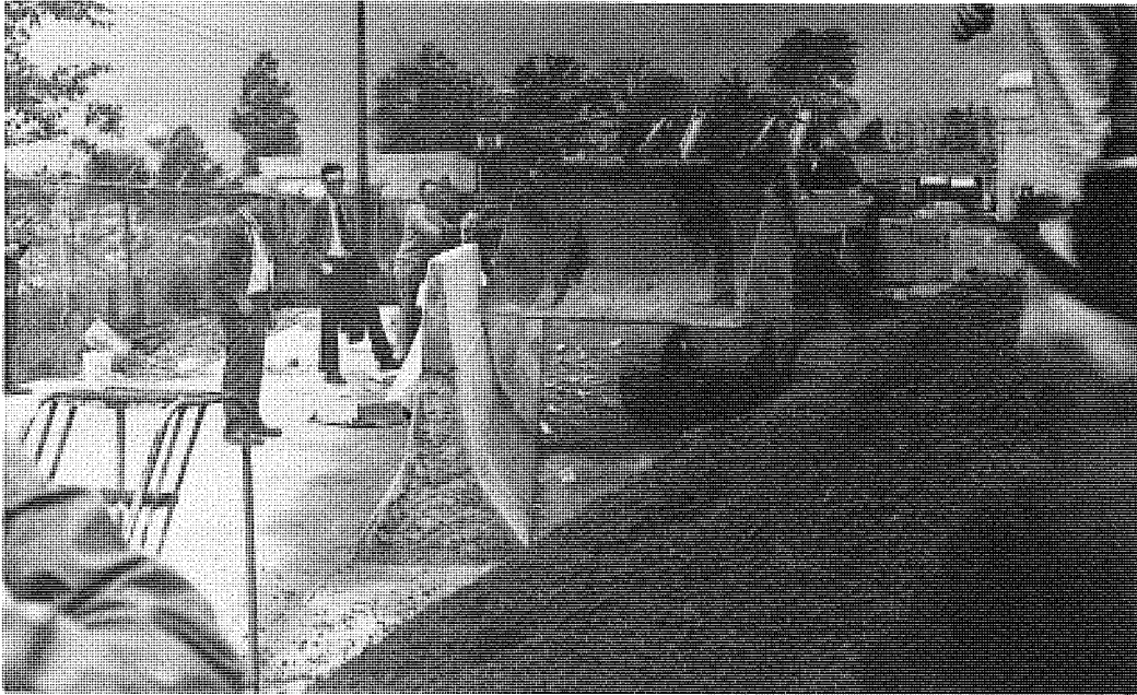
Figure 4. Glare screen being struck by a front-end loader.
