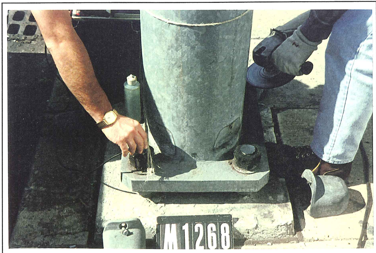
Figure 8 - Ultrasonic Testing of Anchor Bolts for Fatigue Cracks
