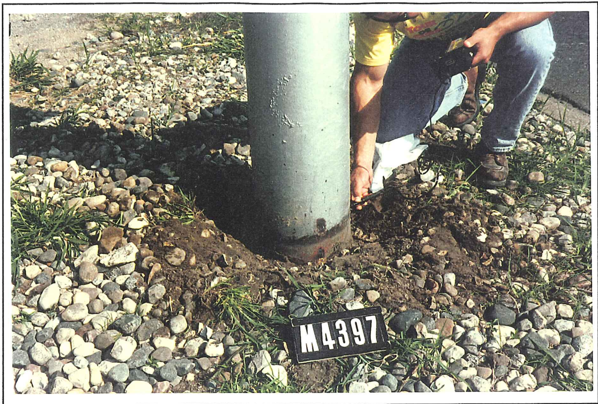
Figure 7 - Ultrasonic Testing to Measure Thickness of Steel Near Base of Pole
