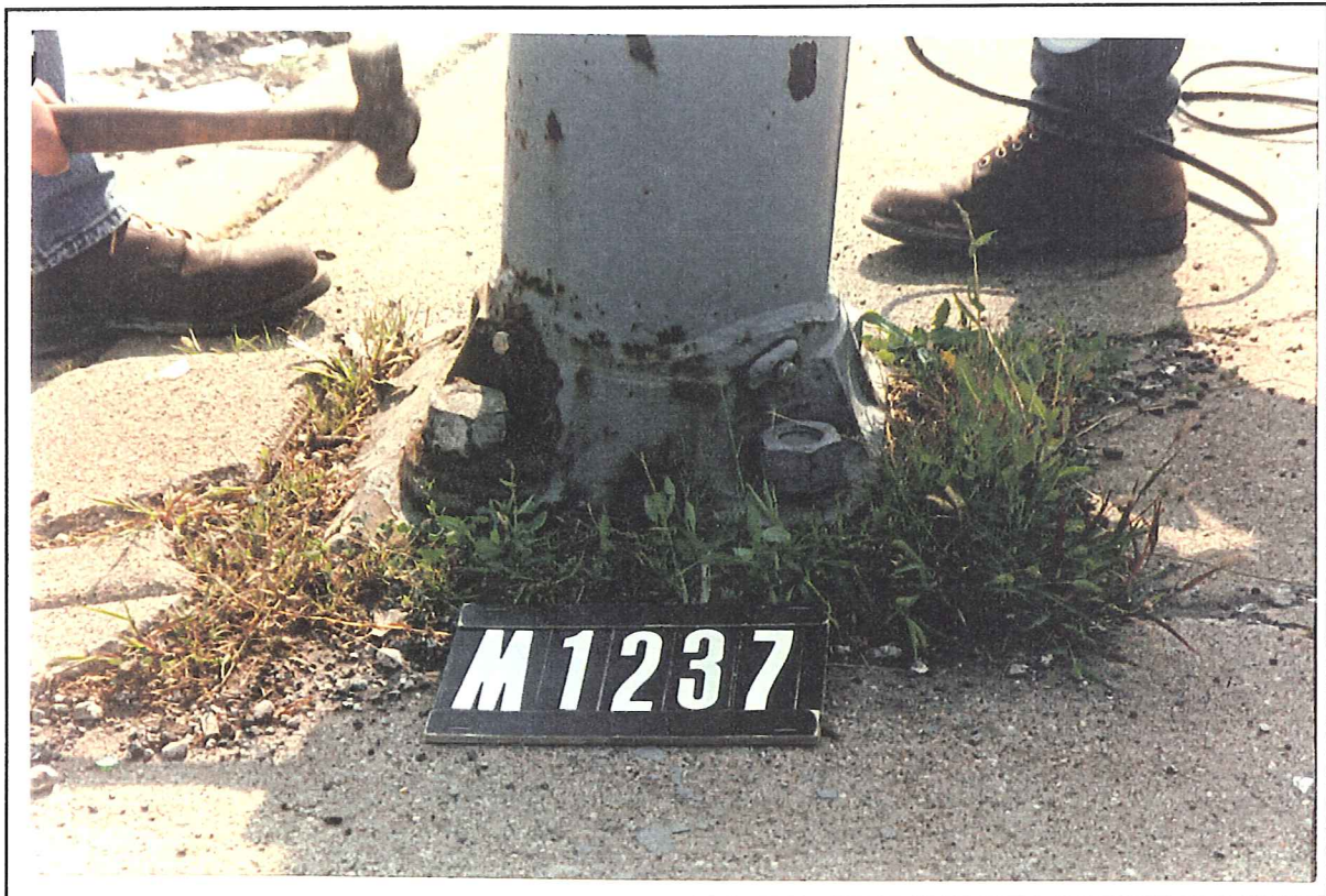
Figure 6 - Hammer Test to Sound Anchor Nuts/Bolts
