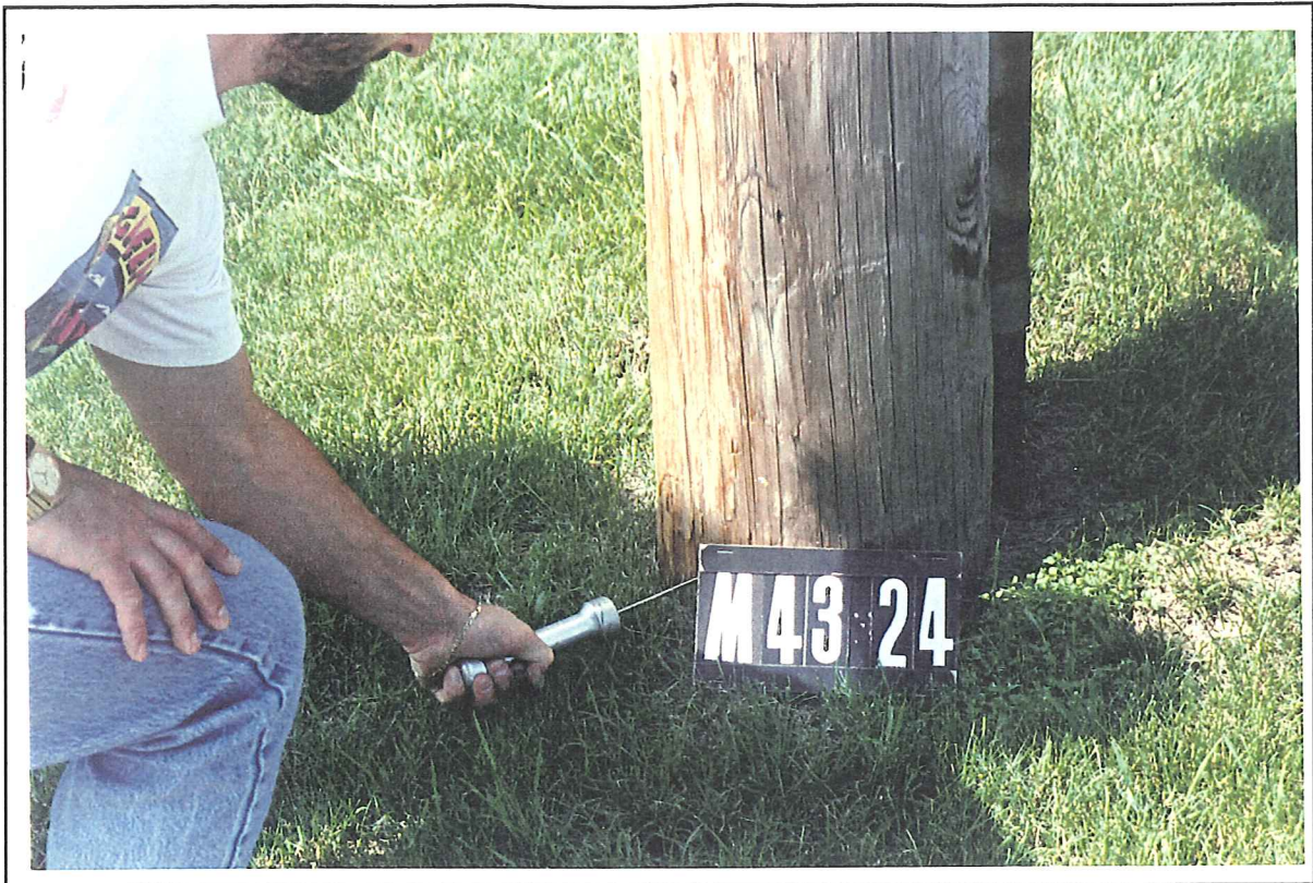
Figure 5 - Probe Test for Soundness of Wood Strain Pole
