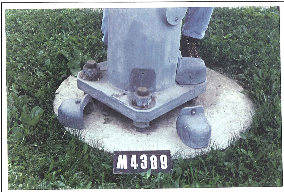
Figure 4 - Typical Galvanized Steel Strain Pole with Raised Base Plate
