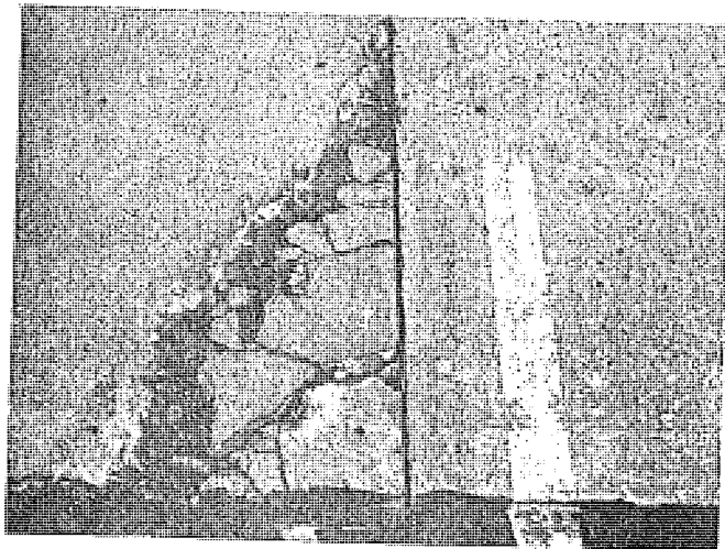
Figure A16. Slab corner spalling, interior.
