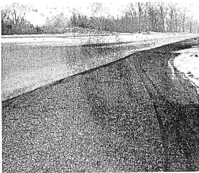
Figure A27. Frost heave. The differential upward displacement of pavement due to action of frost which has caused localized swelling of the subgrade.
