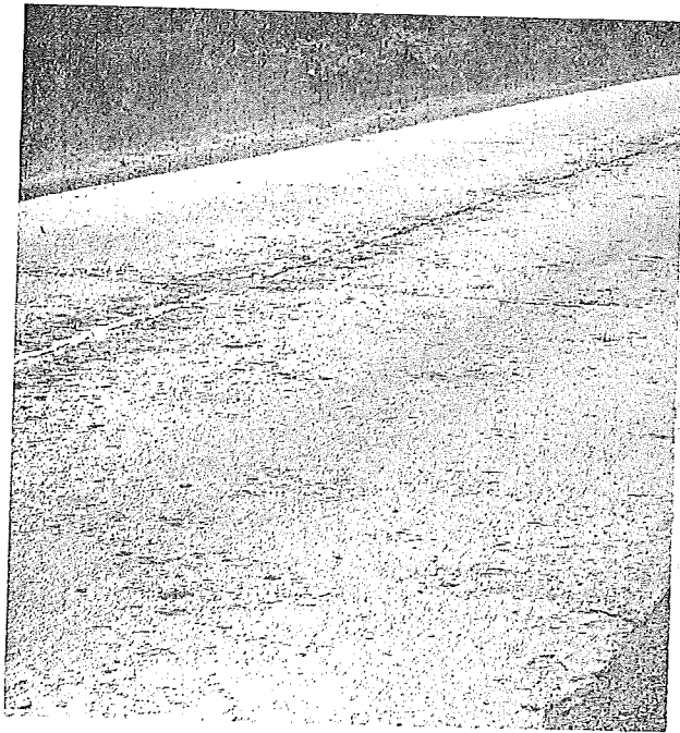
Figure A29. Progressive scale. A condition of concrete disintegration which in its initial stages appears as surface scale, but gradually progresses deeper below the surface stratum. Tapping or drawing a hammer over such areas generally produces a hollow or "plunky" sound.
