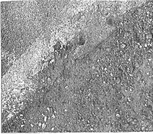
Figure A18. Joint groove spalling.
