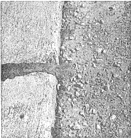
▲ Figure A12. Patch. In an area less than a full lane in width, (a) the covering over with or without removal of the existing pavement, or (b) removal and replacement of all the existing pavement, with portland cement concrete, bituminous concrete, tar and chip mix, or other materials.
