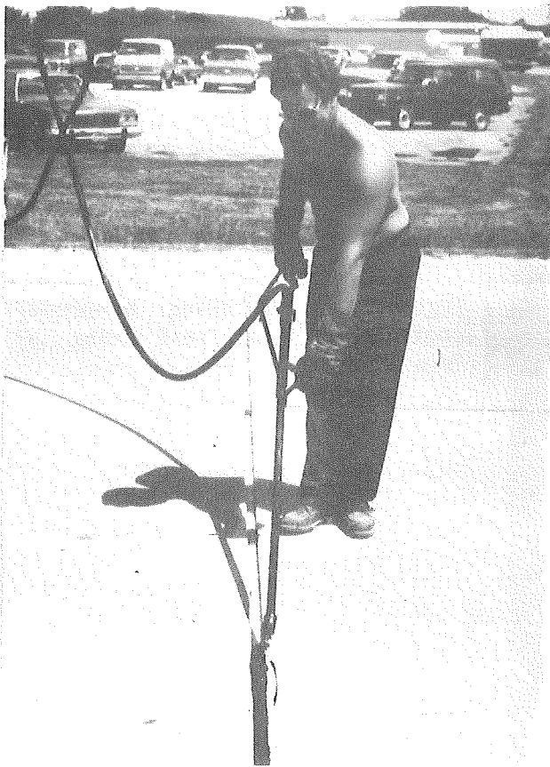
Figure 8. Sandblasted joint groove with foam rod in place.
