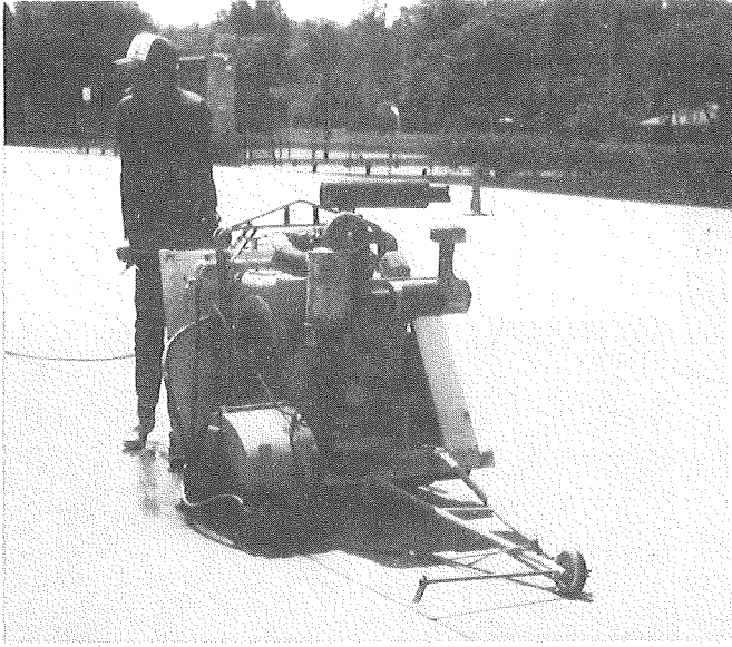
Figure 16. Resawing longitudinal joint groove.
