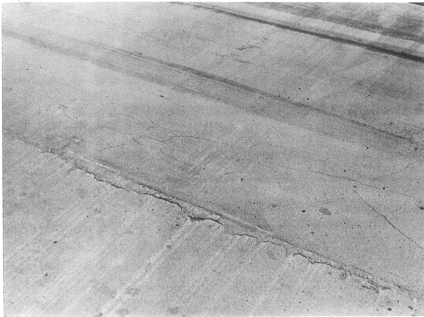
Figure 11. Cracking and loose mortar in west end of Lane D after one winter. April 1958.
