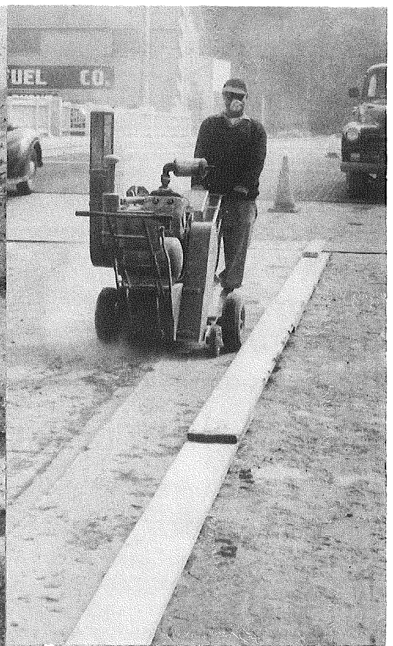
Figure 4. Cutting machine used to remove minimum of 1/2 in. of scaled concrete.
