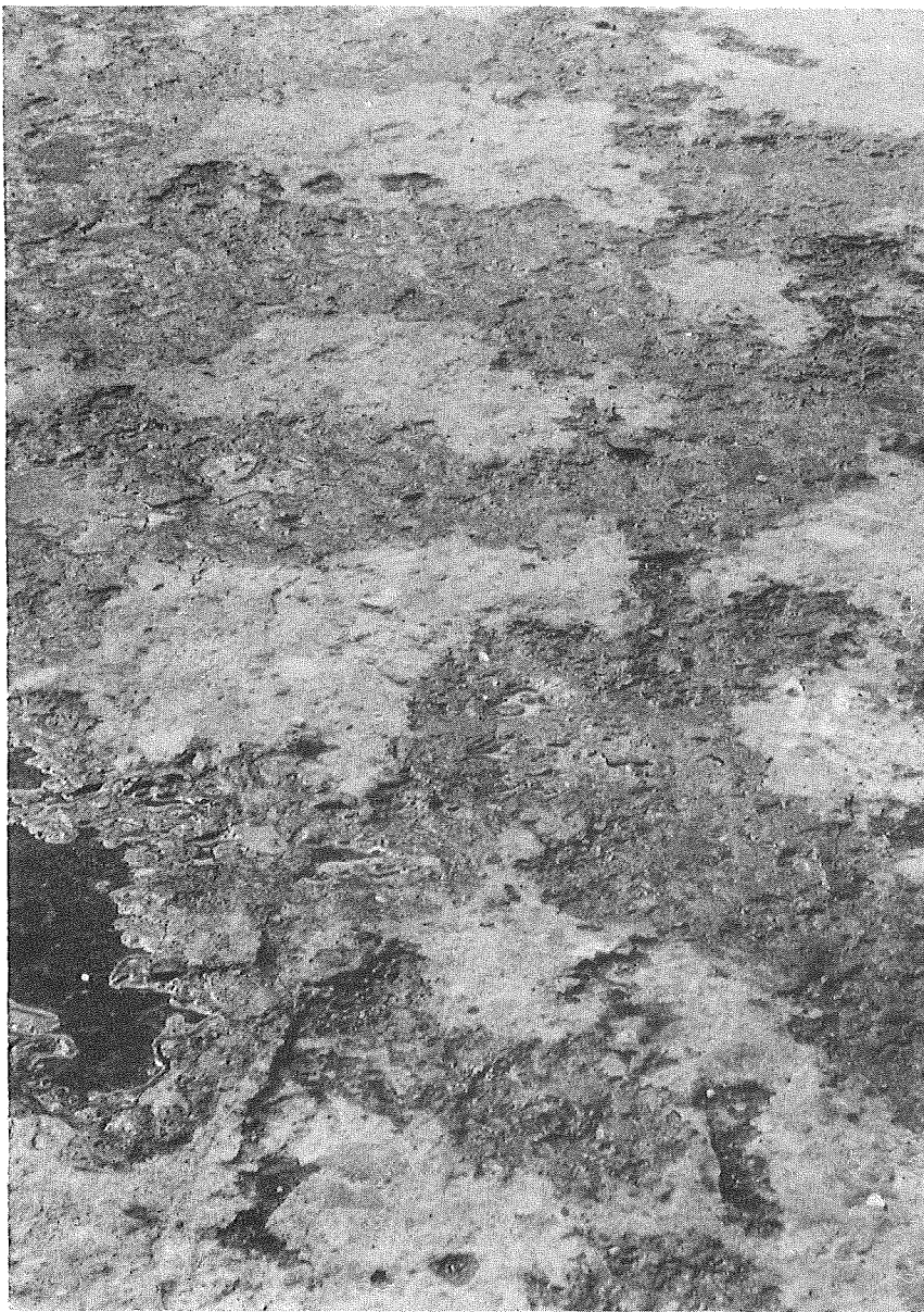
Figure 5. North sidewalk patches chipped to squared edges.
