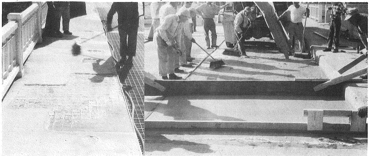
Figure 5. North sidewalk patches chipped to squared edges.
