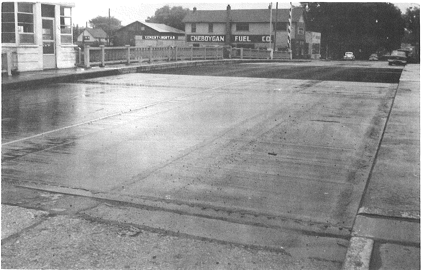
Figure 16. General views of the bridge deck showing overall sound condition of latex mortar lanes in August 1959, after two winters; east end (top) and west end (bottom).
