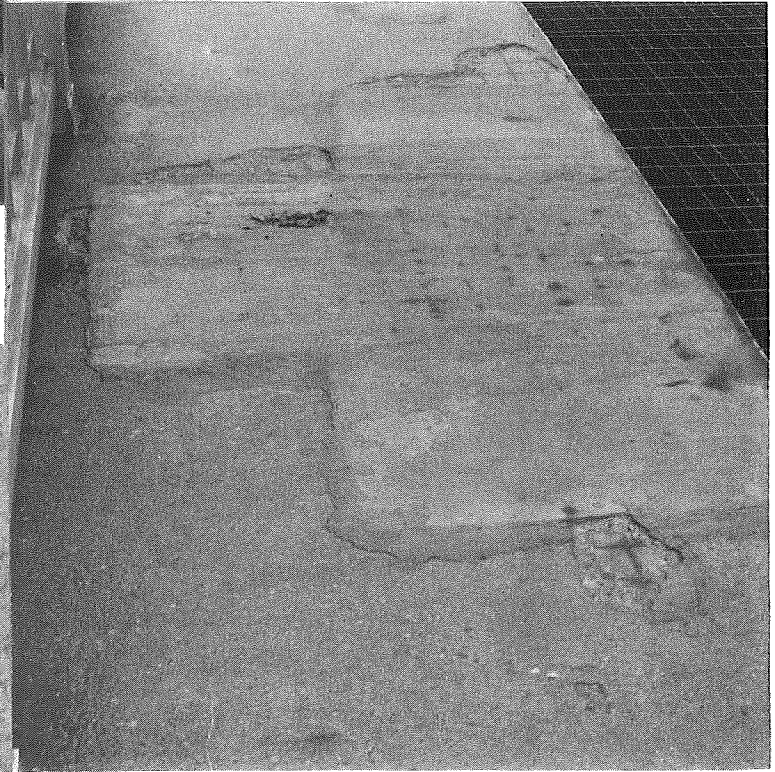
Figure 14. Further failure around large latex mortar patch in north sidewalk.
