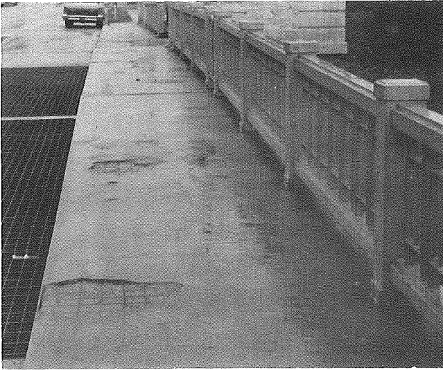
Figure 13. Newly spalled areas in north sidewalk, some adjacent to patches.
