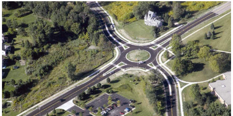
One of the almost 100 roundabouts constructed in Michigan since 1996, this roundabout is near Bennett Woods Elementary School at the intersection of Bennett and Hulett roads in Okemos.
