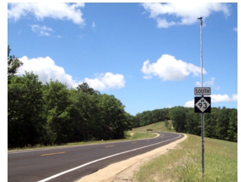
This camera, temporarily mounted on a road sign on a horizontal curve, monitors vehicle position within the lane of traffic and encroachments into the adjacent lane or shoulder.
