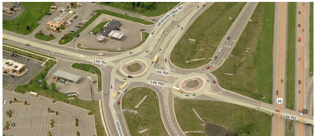
This dual roundabout in Brighton is located at Lee and Whitmore Lake roads and Lee Road and southbound U.S. Highway 23.
