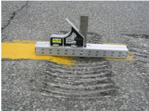
Centerline rumble strips have been shown to reduce cross-centerline crashes.
