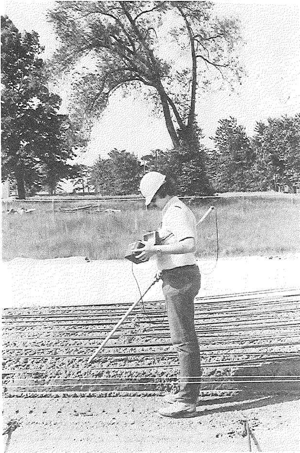
(a) Acoustic probe inserted in concrete and signal being read on control box.
