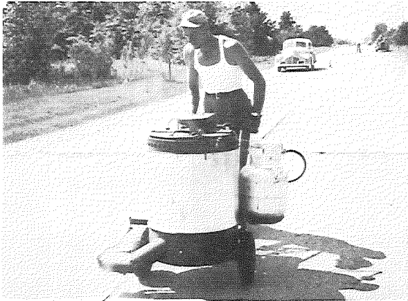
FIGURE 2. SEALING LONGITUDINAL JOINT WITH MECHANICAL POURPOT.
