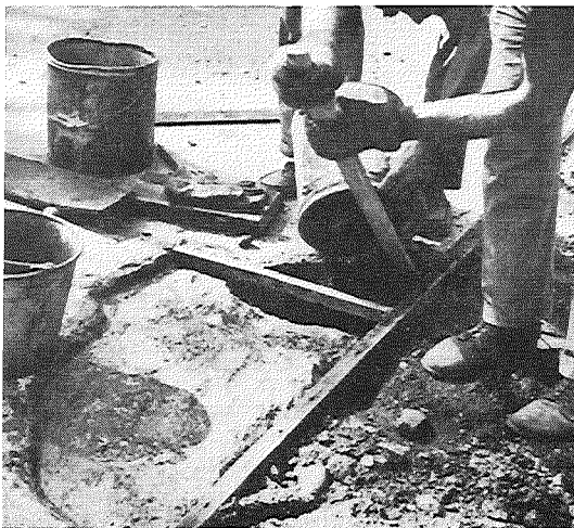
▼ FIGURE 15. ADDING GROUTING MIXTURE.
