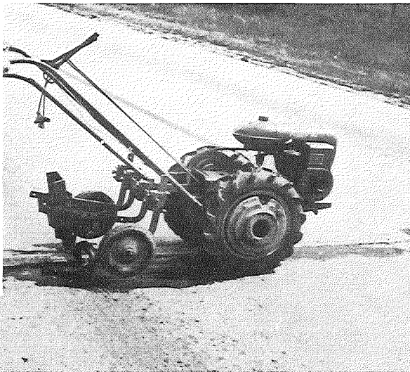
FIGURE 6. GARDEN TRACTOR WITH PLOW ATTACHMENT REMOVING OLD JOINT SEALER.
