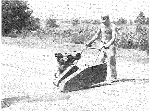
FIGURE 3. CONTRACTOR'S JOINT - CLEANING MACHINE IN OPERATION.
