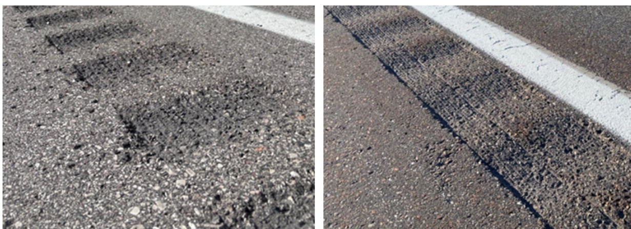
Traditional Rectangular (left) and Sinusoidal (right) Shoulder Corrugations
