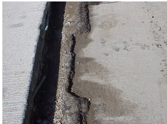
Figure 6. Asphalt separator layer broken from paver track.
