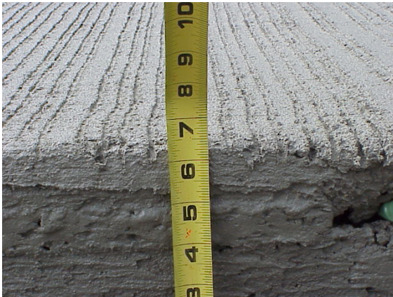
Figure 10. Concrete overlay close to the six inch proposed thickness.
