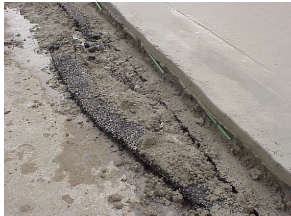
Figure 6. Asphalt separator layer broken from paver track.
