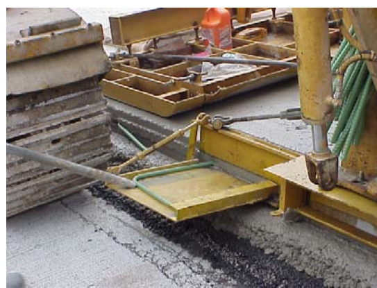
Figure 3. Set-up for placing tie bars at edge of paver.
