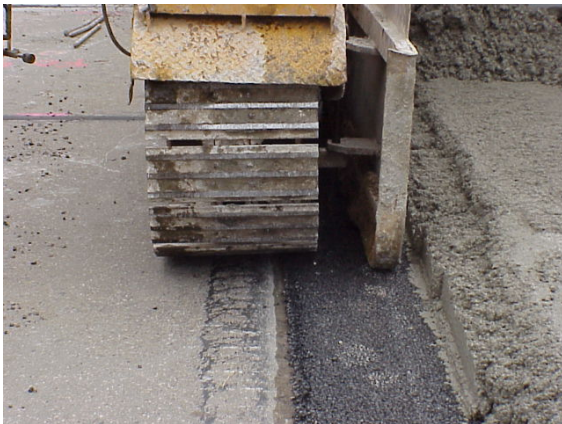
Figure 5. Paver track running on asphalt separator layer.
