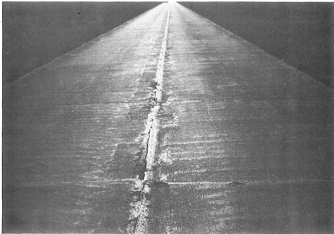
Figure 3. Typical appearance of slippery stone sand concrete surface under reflected light.
