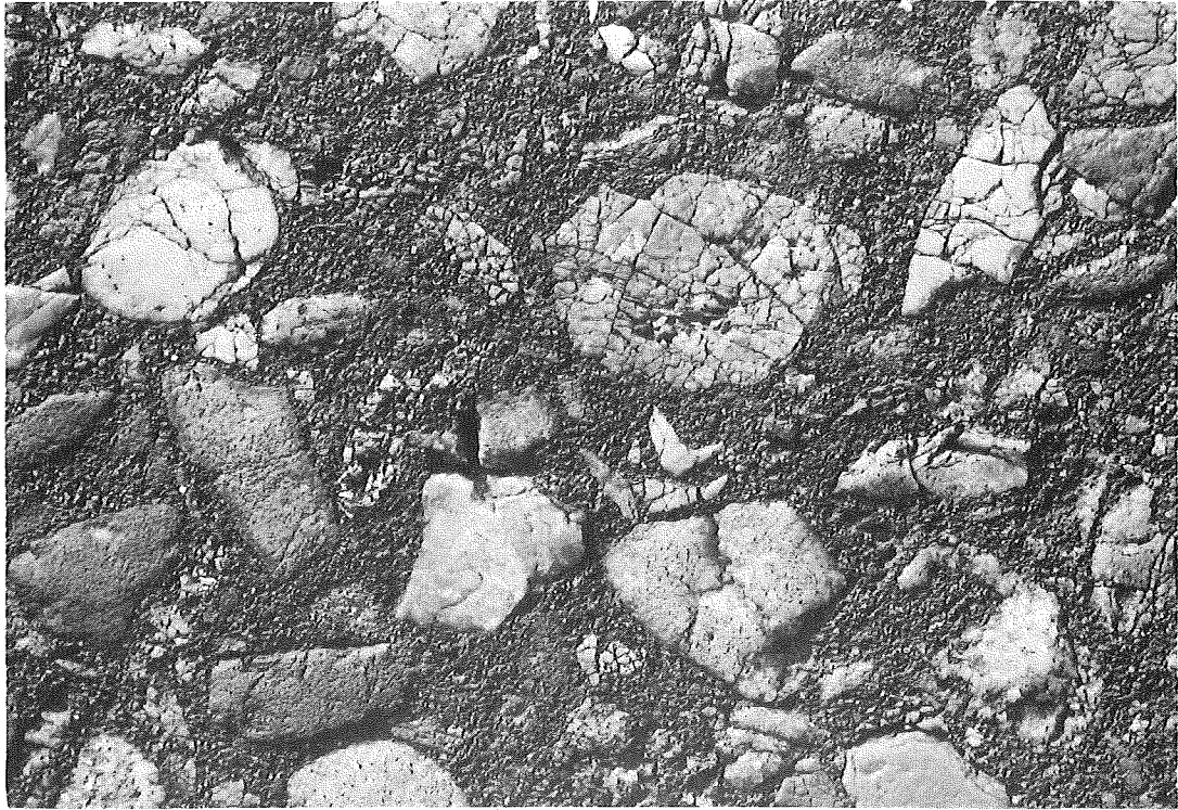
Figure 15. Bituminous concrete gravel aggregate, traffic lane, age 4 years; Coef. 0.55, average daily traffic 3120.
