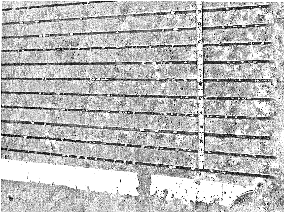
Figure 4. Transverse grooved concrete, eastbound temp I 69 at M 52, Perry.
