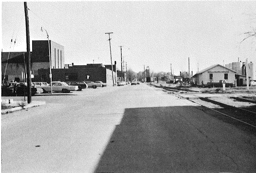
EASTBOUND ADAMS STREET
