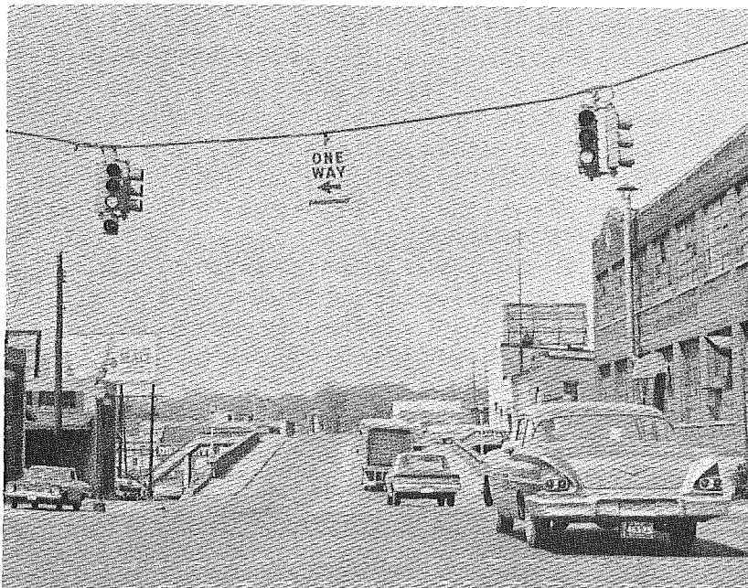
Figure 4-3. Traffic control signal installation with delayed left turn arrow.
