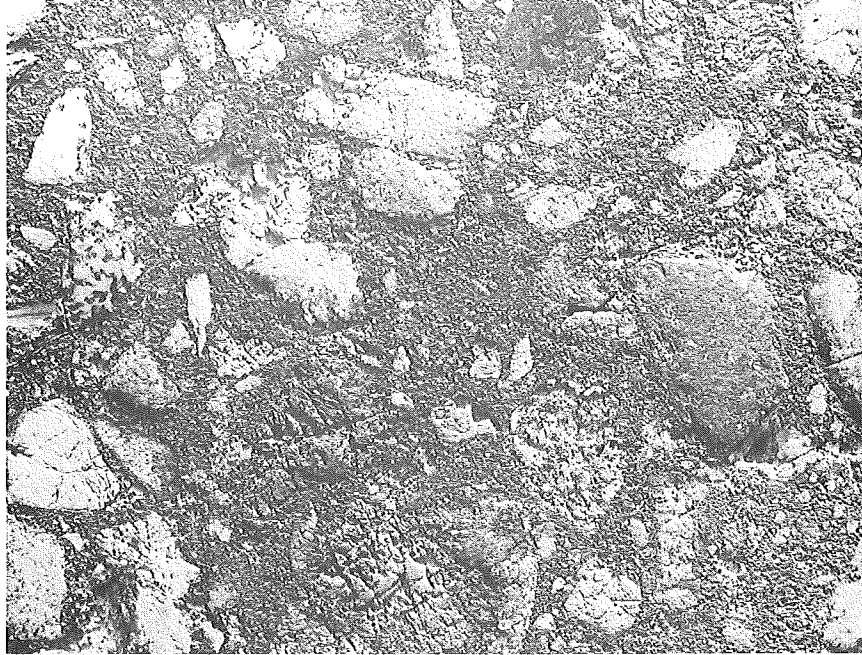
Figure 20—Project 12, Gravel aggregate 25A, Traffic Lane coef. 0.50. Age 3 years. Average daily traffic, 12,000. West end of project. Wear factor 15.5.
