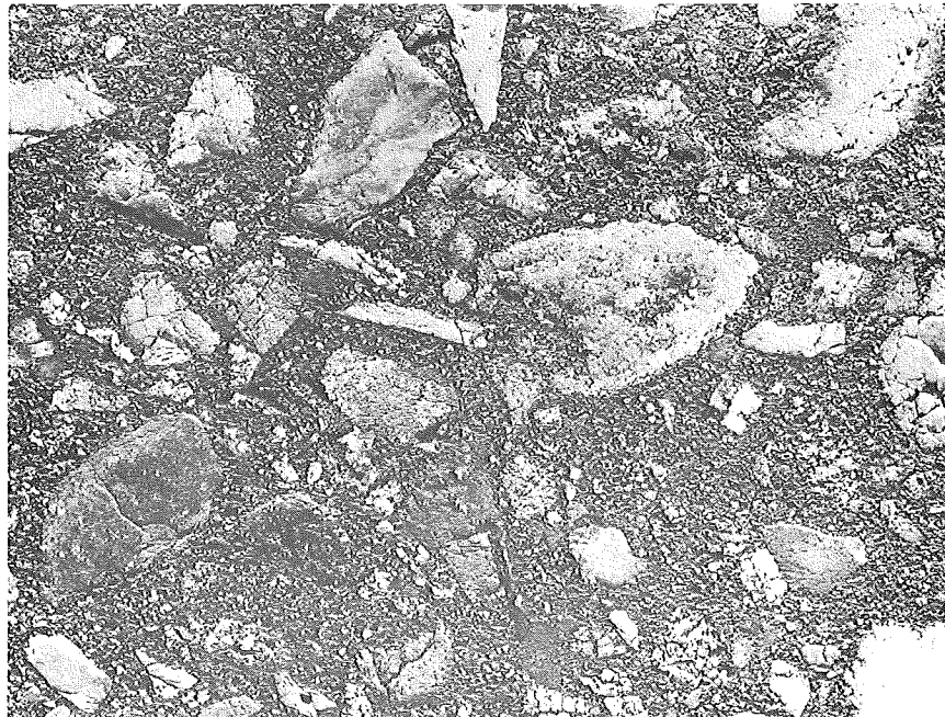
Figure 21—Project 12, Gravel aggregate 25A, Traffic Lane, coef. 0.405. Age 3 years. Average daily traffic, 16,000. East end of project. Wear factor 20.0.
