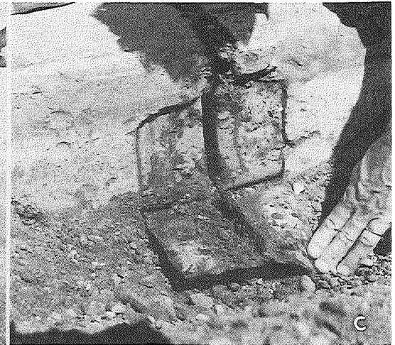
Figure 11. Spalls were observed near the inner edge, near the centerline, and at the outer edge of this joint (A, view from outer edge). Excavation at the outer edge showed fair alignment of the base plate and joint groove (B), with considerable infiltration of foreign material (C). However, excavation at the inner edge (D) showed base plate embedment in the slab concrete. The extreme tilt of the base plate (E) suggests that it may have been moved by paving equipment during pouring or placed on an unlevel base. In either case, the dowel bar assembly may also have been tilted, a possible explanation for the surface spalling. 1392+42; EB; 34044, C1
