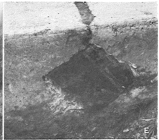
Figure 11. Spalls were observed near the inner edge, near the centerline, and at the outer edge of this joint (A, view from outer edge). Excavation at the outer edge showed fair alignment of the base plate and joint groove (B), with considerable infiltration of foreign material (C). However, excavation at the inner edge (D) showed base plate embedment in the slab concrete. The extreme tilt of the base plate (E) suggests that it may have been moved by paving equipment during pouring or placed on an unlevel base. In either case, the dowel bar assembly may also have been tilted, a possible explanation for the surface spalling. 1392+42; EB; 34044, C1
