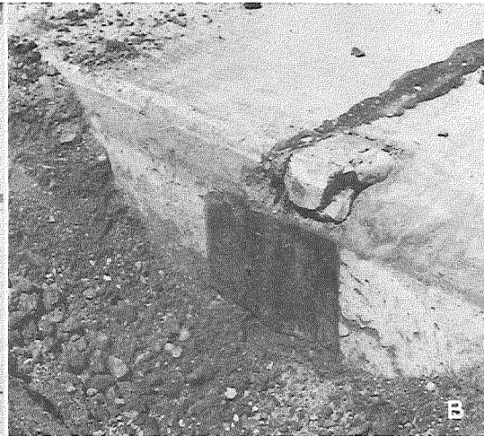
Figure 11. Spalls were observed near the inner edge, near the centerline, and at the outer edge of this joint (A, view from outer edge). Excavation at the outer edge showed fair alignment of the base plate and joint groove (B), with considerable infiltration of foreign material (C). However, excavation at the inner edge (D) showed base plate embedment in the slab concrete. The extreme tilt of the base plate (E) suggests that it may have been moved by paving equipment during pouring or placed on an unlevel base. In either case, the dowel bar assembly may also have been tilted, a possible explanation for the surface spalling. 1392+42; EB; 34044, C1
