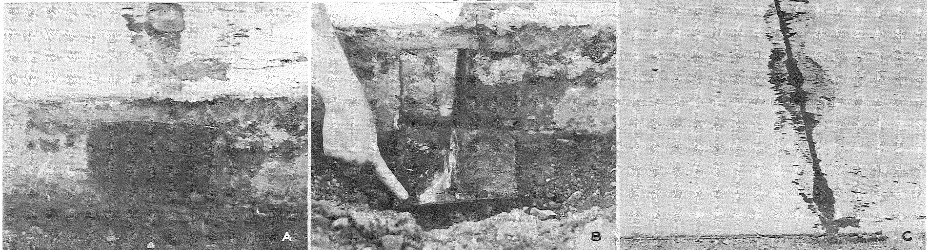
Figure 10. Deterioration along this joint (C) may be related to dowel misalignment, which could also explain the base plate's tilt and misalignment (A). Spalling at this outer slab edge has allowed infiltration of foreign material into the joint (B). 1371+57; EB; 34044, C1
