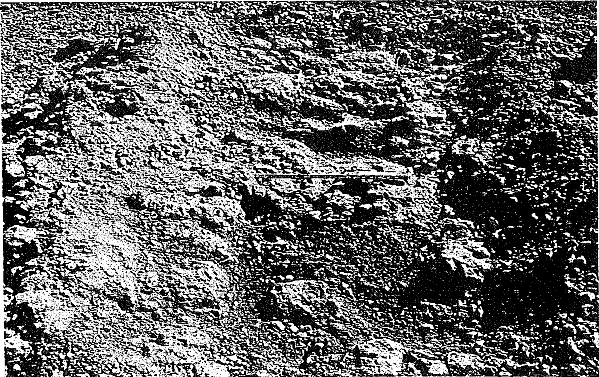
Figure B.24 Portage Road NBIL (Portage) trench in rubblized concrete (station 3+901.5) resonant breaker
