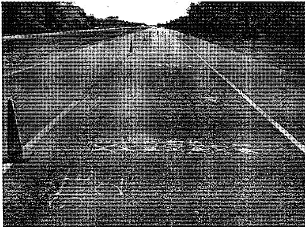
Figure C.3 I-69 EB section test site 2 at mile marker 127
