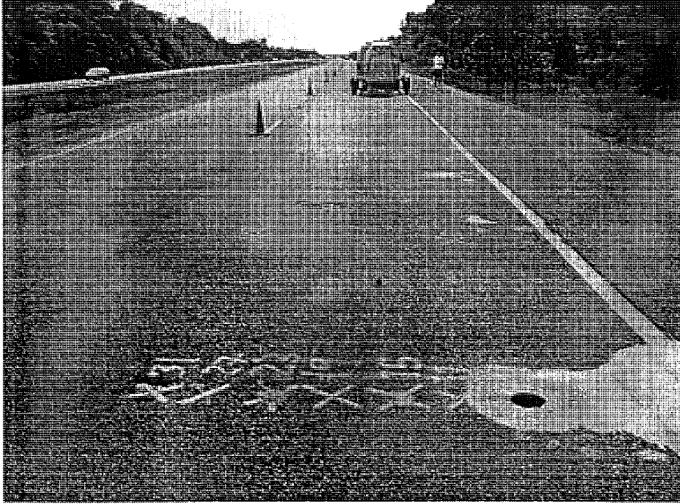
Figure C.2 I-69 EB section test site 1 at mile marker 127
