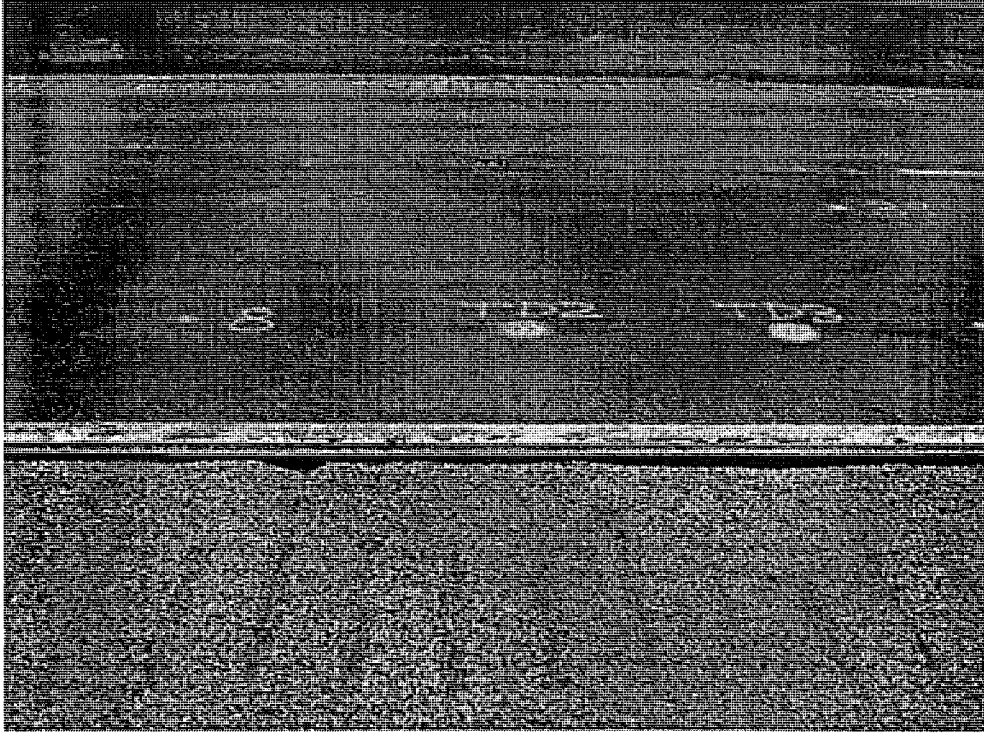
Figure C.19 Cores TD2 and TD3 over an alligator crack on US-27 SB section test site 1
