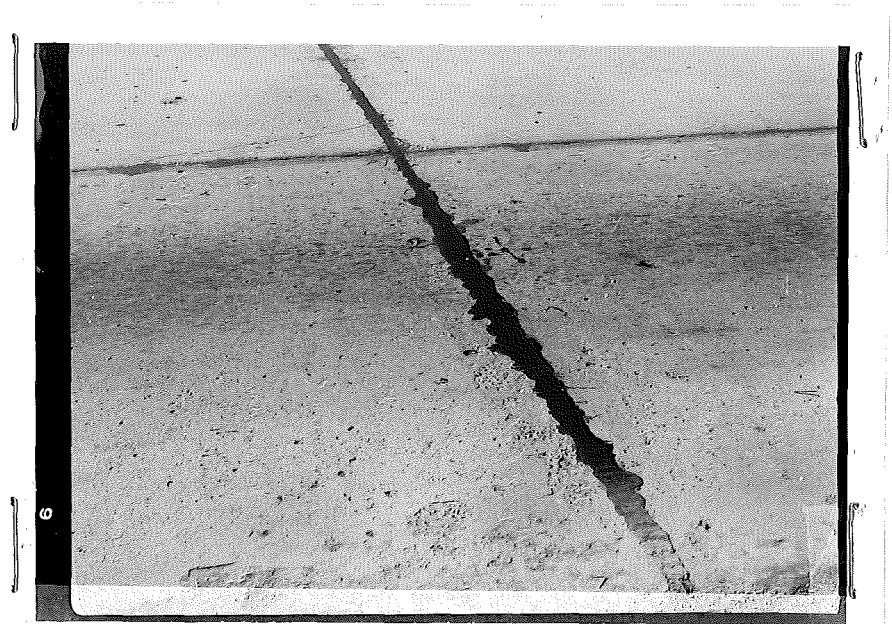
Figure 6. Oil-Anode GRS. North half looking south. Station 184+80. Provides excellent seal, but too soft.
