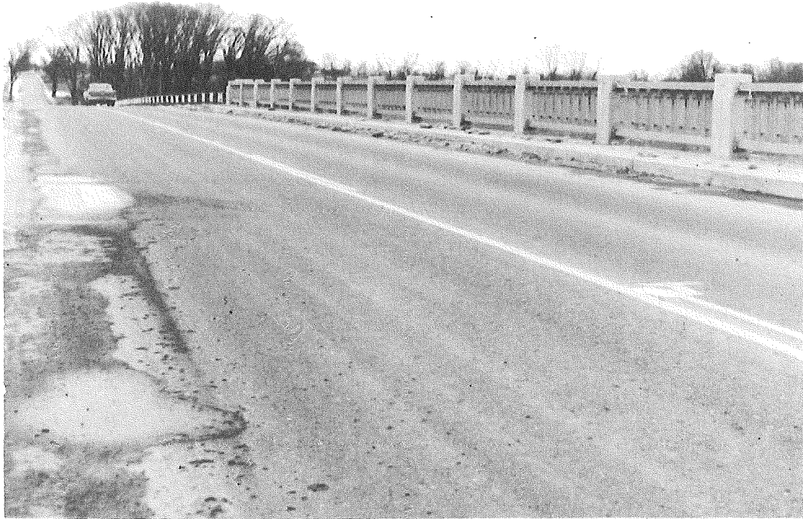
Figure 7. Dettman Road overpass with bituminous aggregate resurfacing (2-60).
