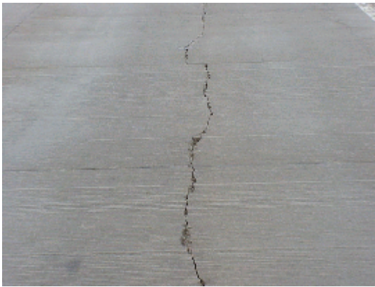
Figure 6. Closer Look at the Spalling
