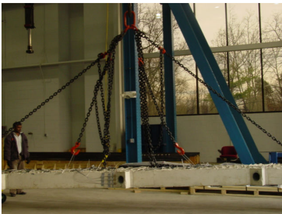
(a) Box-beam lifted using crane
