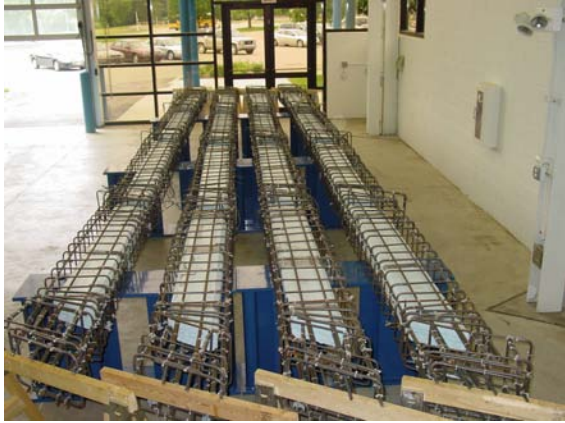
(a) Reinforcement cages for the box-beams
