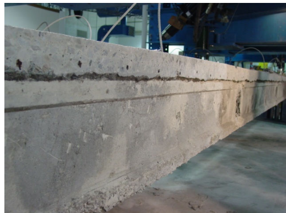
(b) Grout removed from shear-key
