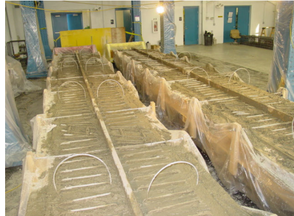
(b) Casted box-beams
