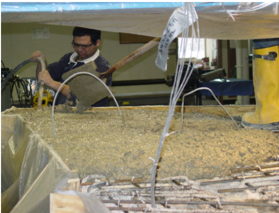
(a) Casting of deck slab for the bridge model
