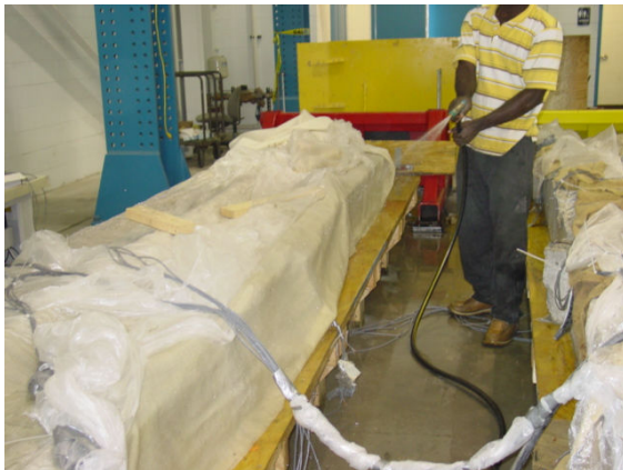
(c) Wetting of burlap for curing
