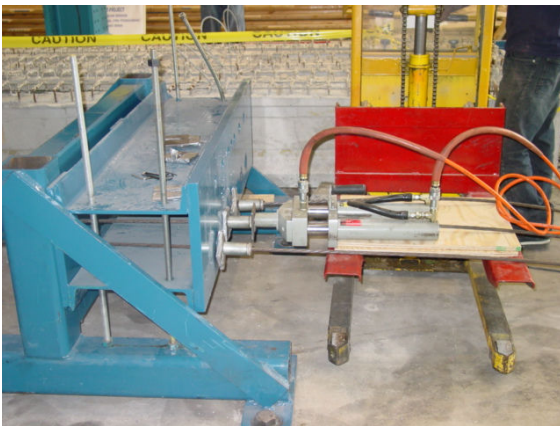
(c) Pre-tensioning of steel strands
