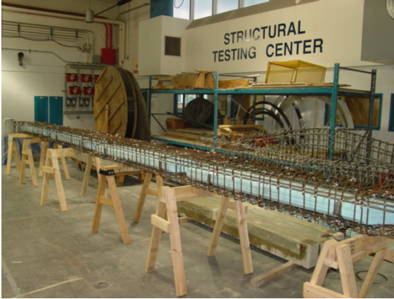
(a) Construction of steel cages
