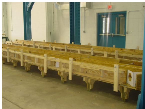
(a) Side view of formwork
