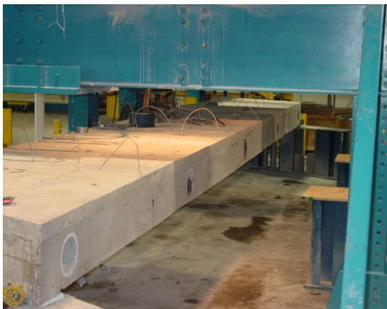
(a) Remained portion of shear-key
