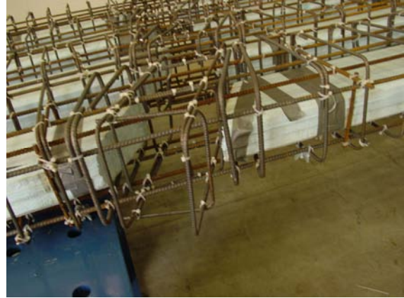
(b) Diaphragm reinforcement details
