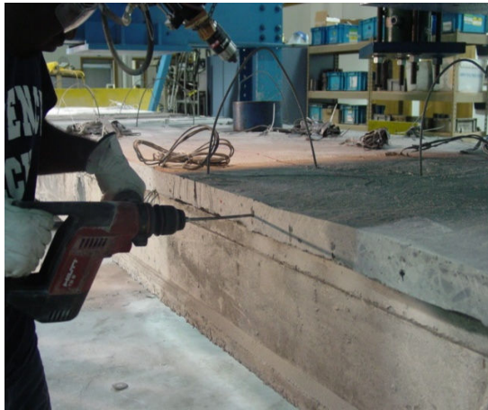
(a) Drilling of horizontal holes
