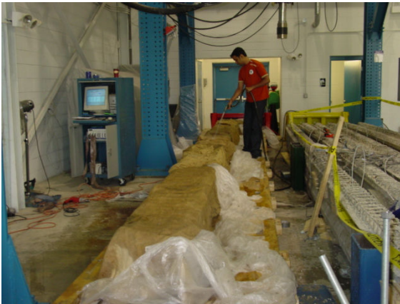
(e) Curing of box-beam
