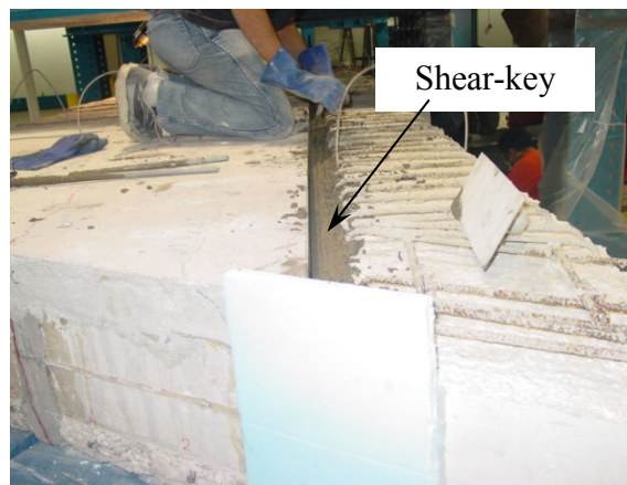
(b) Grouting of new shear-key
