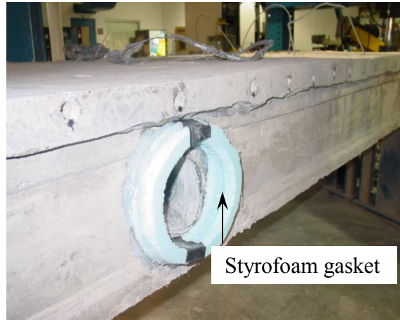
(b) Installation of styrofoam gasket
