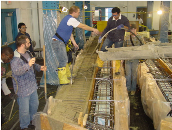
(a) Vibration of concrete for exterior beam
