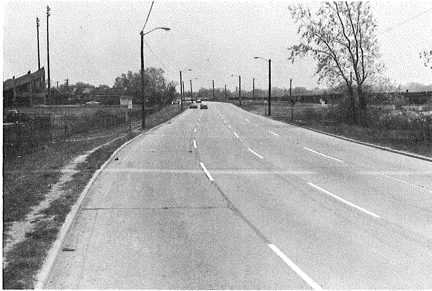
PONTIAC: Four-lane section of one-way Cass Avenue looking southeast
