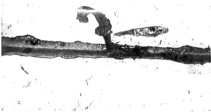
FIGURE 16. JOINT SEALED BY SARGENT CONSTRUCTION COMPANY. ADHESION GOOD BUT NOT PERFECT.
