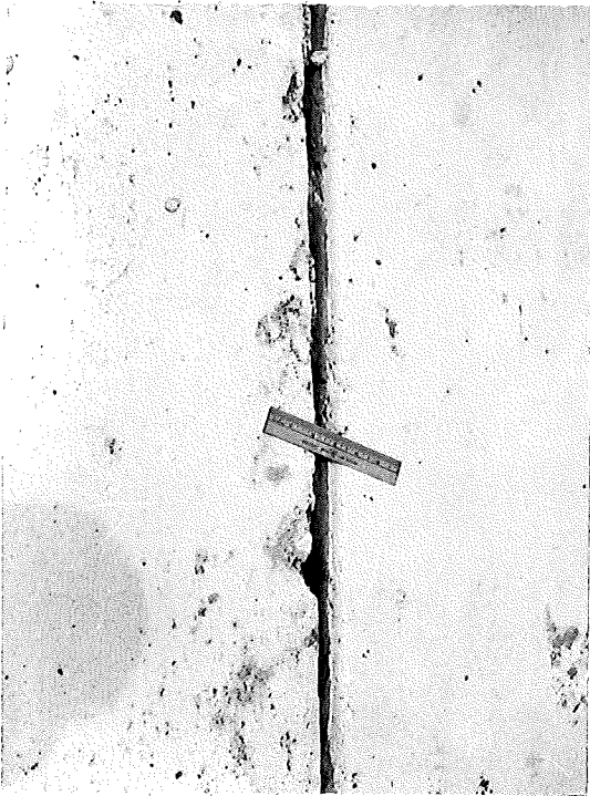
▲ FIGURE 9. MEMBRANE CURING COM- POUND ON JOINT FACE PRIOR TO SEALING BY CARL GOODWIN AND SONS .
