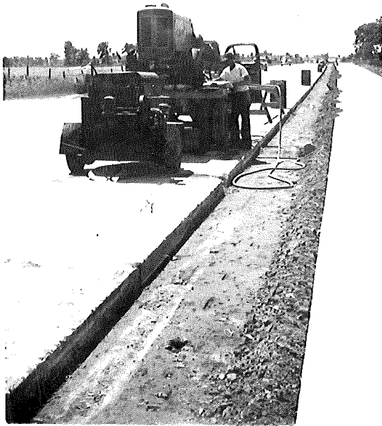
FIGURE 12. JOINT SEAL MELTER AND AIR COMPRESSOR OF SARGENT CONSTRUCTION COMPANY.
