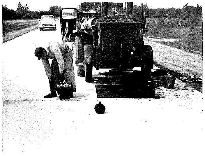
▲ FIGURE 8. JOINT SEAL POURING OPERATION OF CARL GOODWIN AND SONS .
