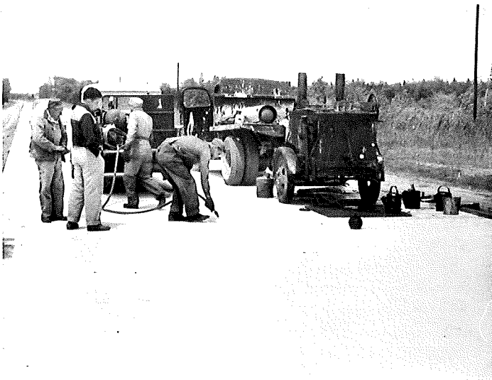
▲ FIGURE 7. JOINT SEAL MELTER, RIGHT, AND AIR BLOWING OPERATION, LEFT, OF CARL GOODWIN AND SONS, CONTRACTORS.
