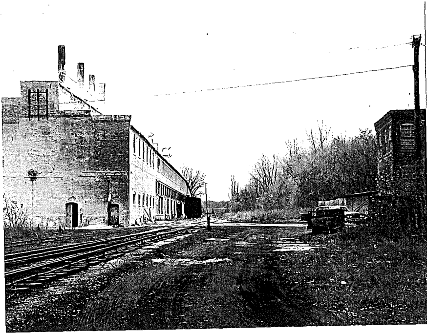
Figure 2. Four stacks on calcining building of Grand Rapids Gypsum Co.
