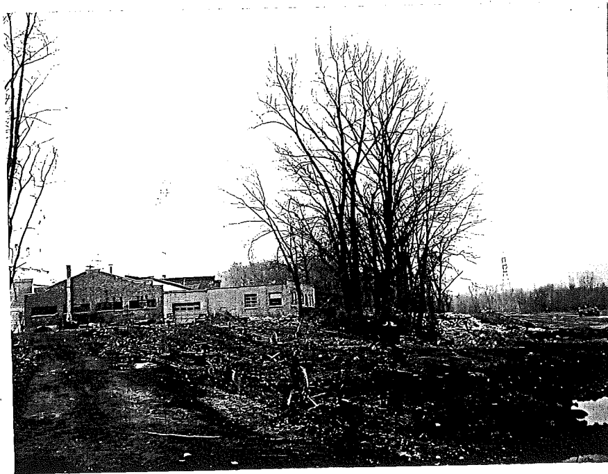
Figure 3. Area southwest of calcining building near I 96 grading operations.
